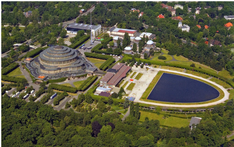
Figure 1: Present-day aerial view of Wroclaw Dome and surroundings
