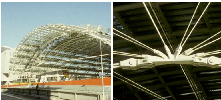
Figure 2: The steel rod structure of the bus terminal in Chur
