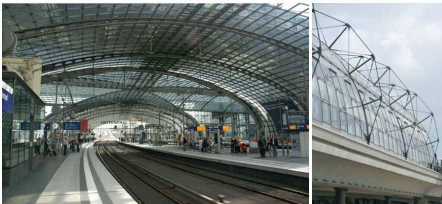
Figure 4: Berlin Hauptbahnhof, its vault and the stabilising undulating rod structure
