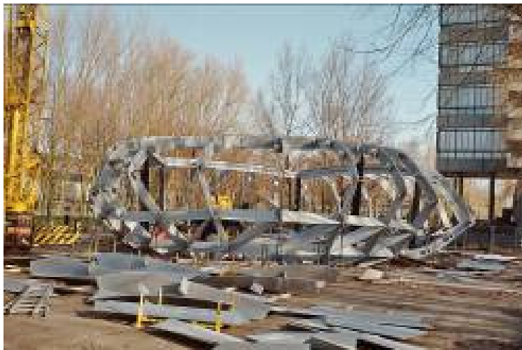
Figure 20: Rebuilding the I-Web at the campus of Delft University.
