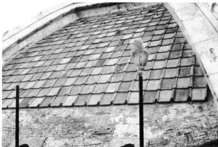
Figure 6: Curved bricks rows emerging under the horizontal tiles rows[7]
