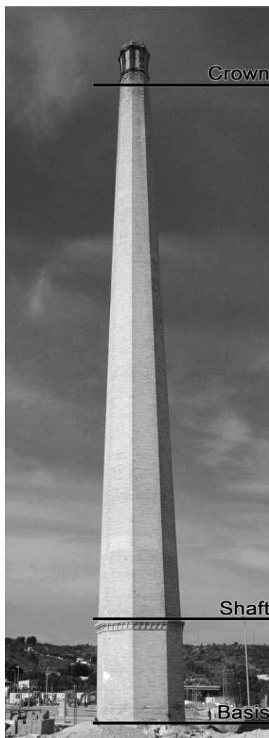
Figure 1. General configuration of an industrial chimney. Chimney factory Aparici, Alcudia de Crespins (Valencia) (Photo: author)
