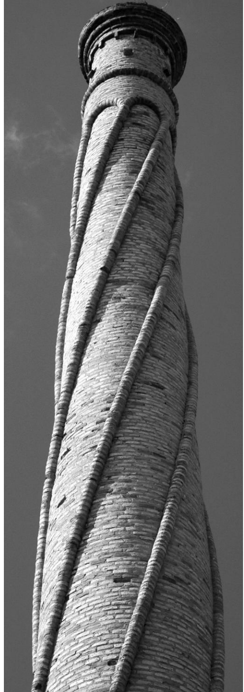
Figure 7. Chimney at the Francisco Isla winery, Villarta de San Juan (Ciudad Real) built by Atilano Millas in 1952. (Photo: author)
