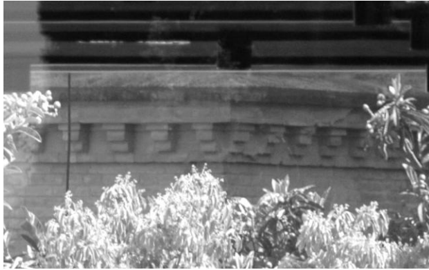
Figure 24. View of the cornice corner of the Martinet Mill chimney, Paterna (Valencia) (Photo: author)
