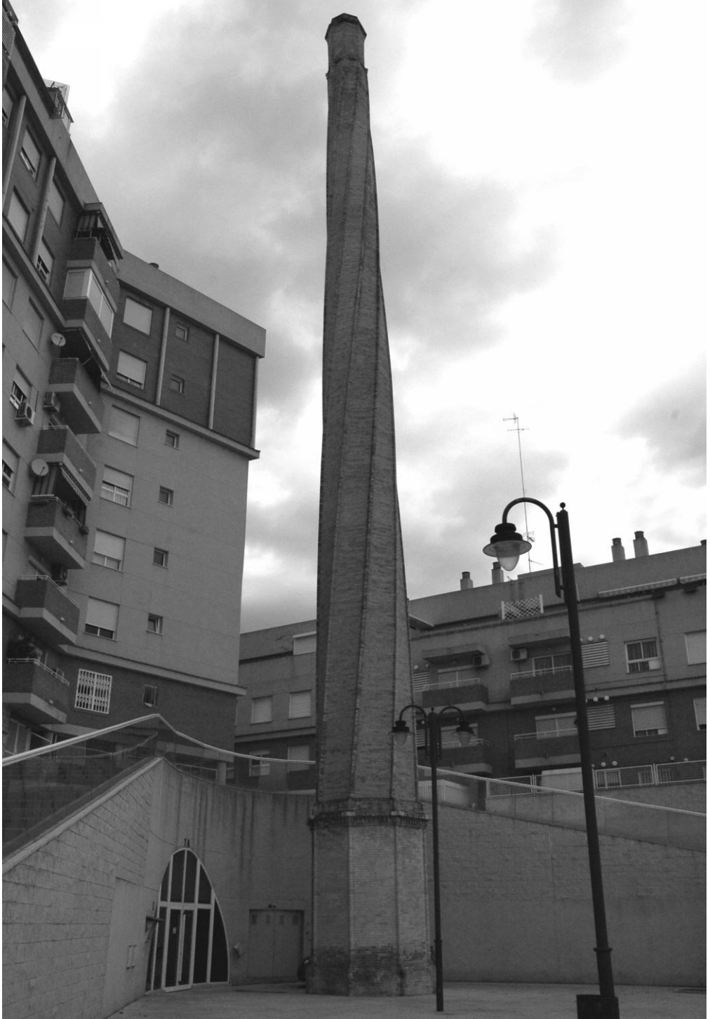
Figure 16. Chimney La Constructora by Agustin Goig, surrounded by residential buildings, Alzira (Valencia) (Photo: author)
