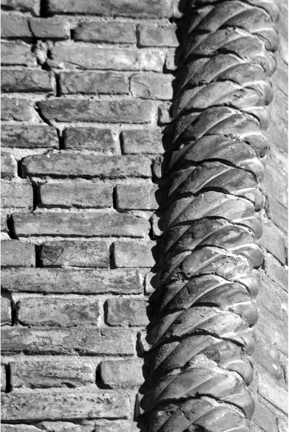
Figure 17. Detail corner cord paper chimney Layana, Valencia (Photo: author)
