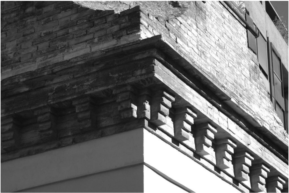
Figure 13. Detail of the corner with modillions in Layana chimney, Valencia (Photo: author)
