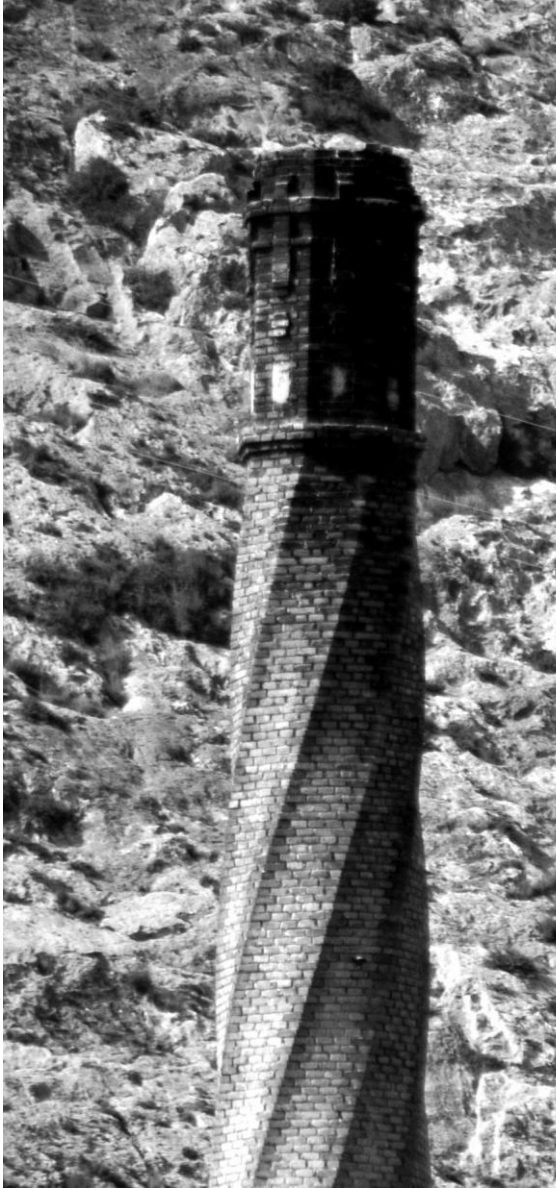
Figure 19. Cooperativa vínico- alcoholera Villenense chimney, Villena (Alicante), 1926 (Photo: author)
