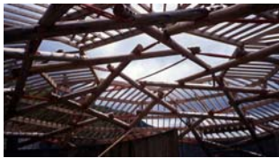
Figure 8 The roof under construction
