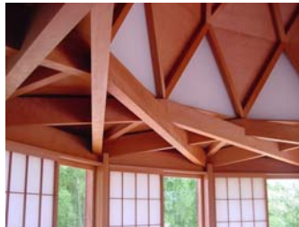
Figure 3 Interior view to Sukiya Yu showing the RF structure
