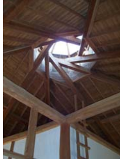
Figure 9 The New Farmhouse building – internal view
