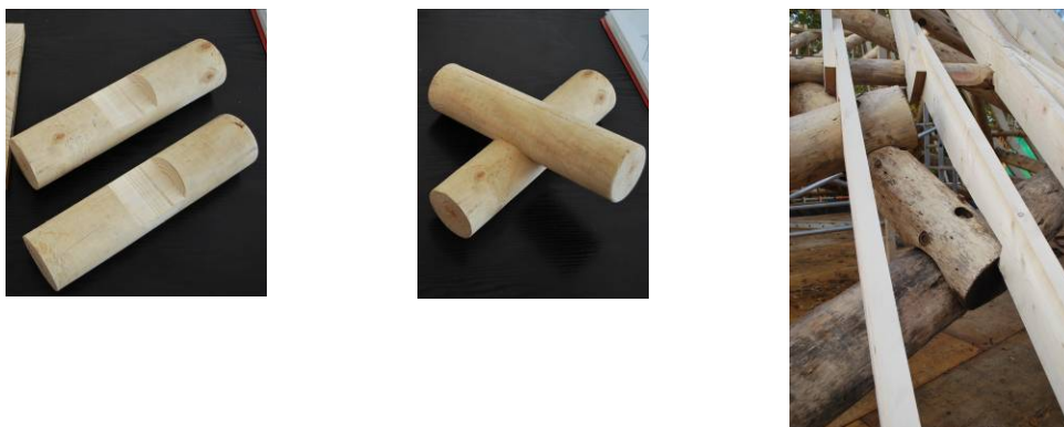
Figure 4: Simple lapped joint with a mainly concealed mechanical fixing: model (left/centre) and actual structure (right). [Photographs: John Chilton]
