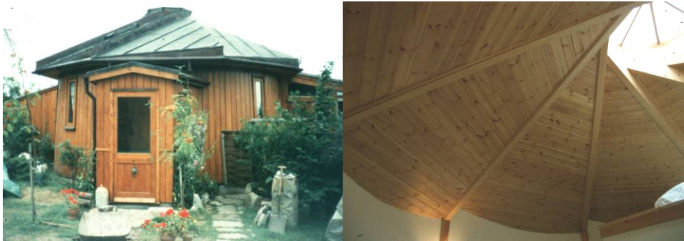
Figure 1: External (left) and internal (right) views of one of the Whisky Barrel Houses at Findhorn Foundation, Scotland (1990). Photographs: John Chilton
