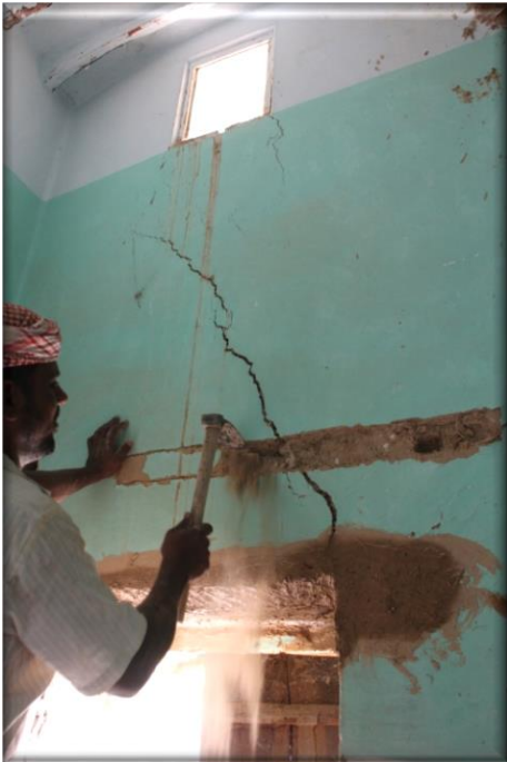
2. Cutting a deeper section to provide hooks.
