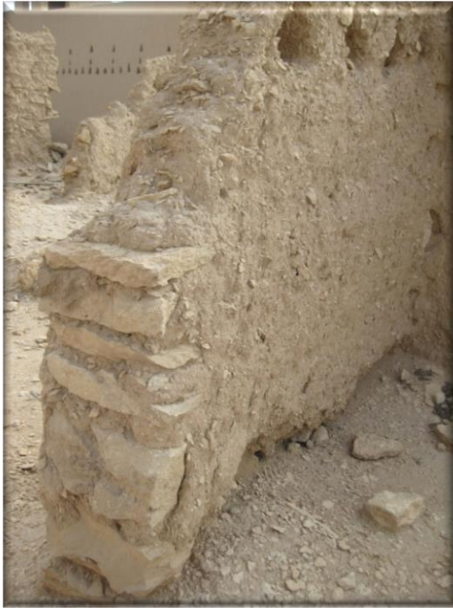
Figure 25. Limestone foundations (Al-Aidarous,2013)
