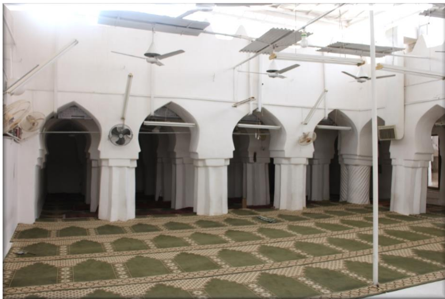
Figure 54. Arches at the Ba-A'alawy Mosque built in adobe (Al-Aidarous,2014)
