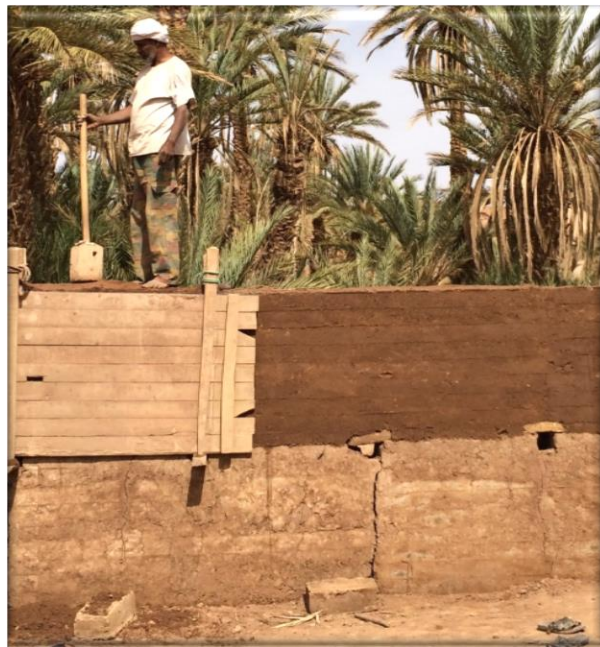
Figure 83. Rammed earth natural rendering (Al-Aidarous,2014)
