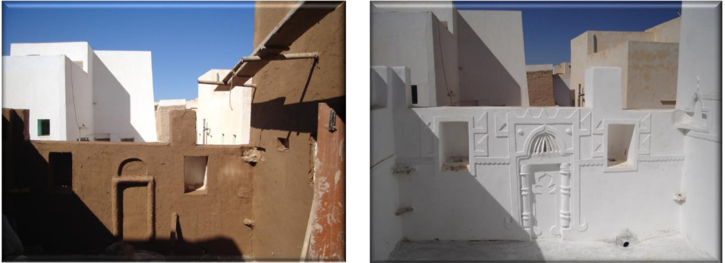
Figure 99. Lime rendering in Hadhramaut (Al-Aidarous,2014)
