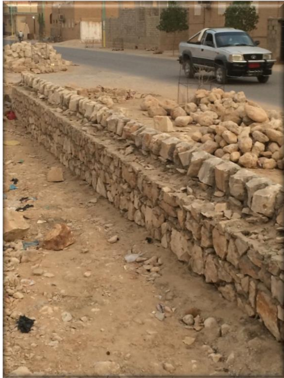
Figure 63. Foundation and thickness of walls (AL-Aidarous,2014)
