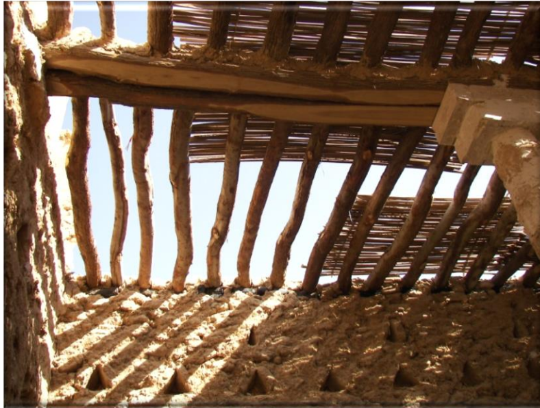
Figure 87. Roof construction (Al-Aidarous,2013)
