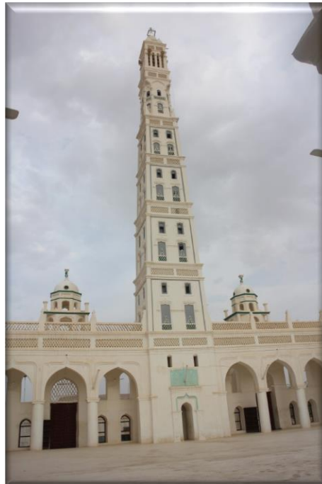
Figure 67. Al-Mehdar Mosque (Al-Aidarous)
