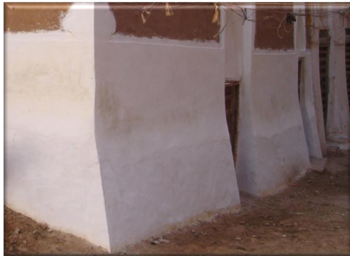
Figure 93. Foundation restoration (Al-Aidarous,2014)
