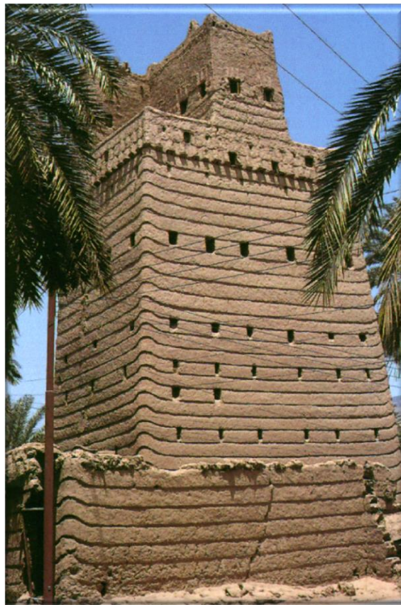
Figure 33. Model of Asir cob house in Najran (Murtadah)
