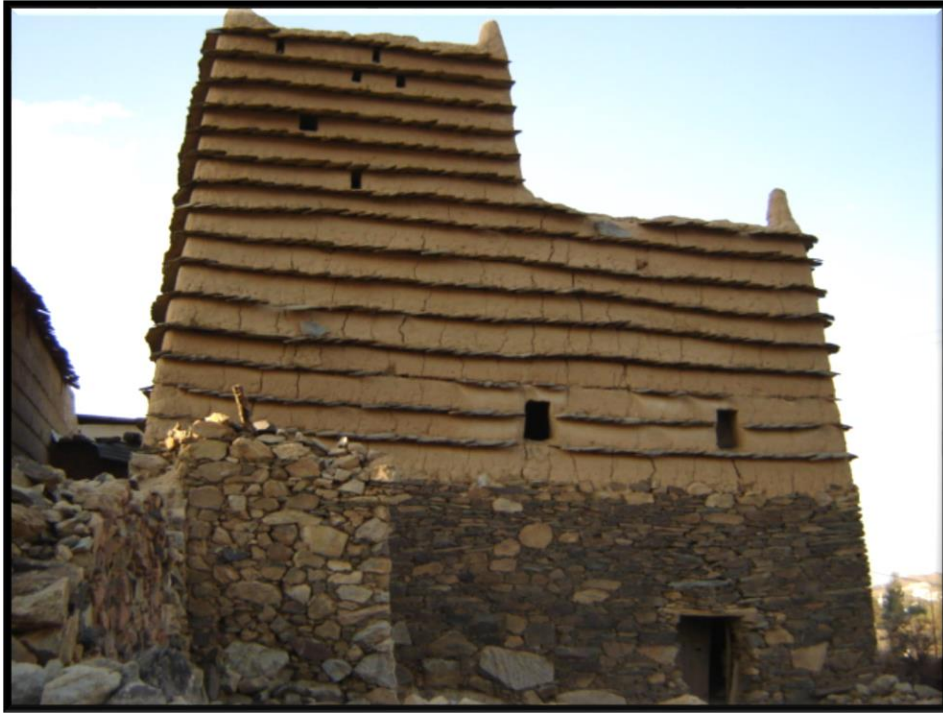
Figure 35. Asiri cob house with horizontal bands of slabs (Murtadah)
