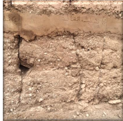
2. Remove all powdery material
