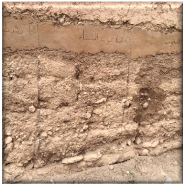
3. Making the mortar
