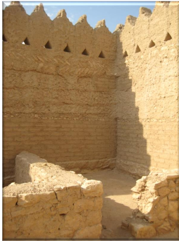
Figure 22. Limestone foundation (Al-Aidarous,2013)
