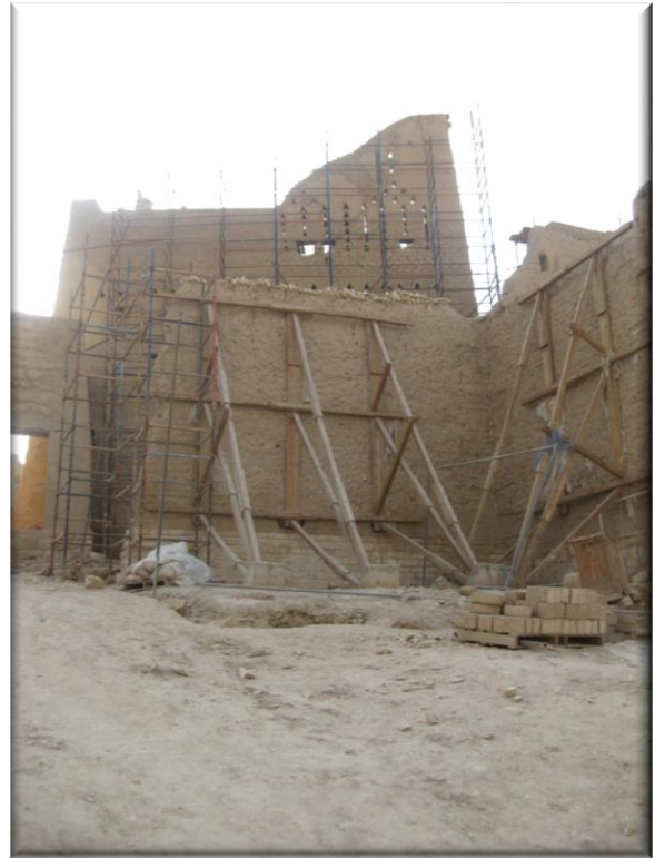
Figure 92. Reinforcement of a structure in ad-Dir'iyah (Al-Aidarous,2013)
