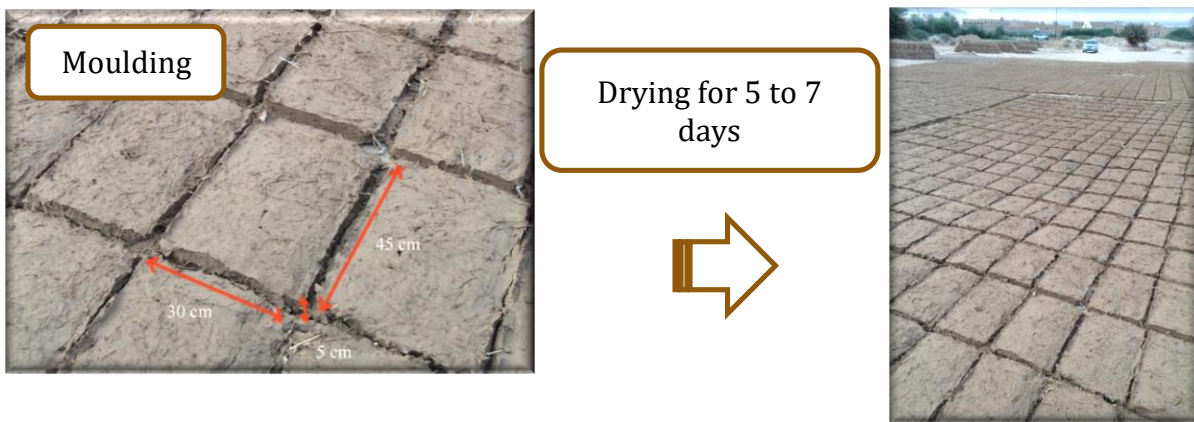
Figure 70. Process of making the adobe (Al-Aidarous,2014)
