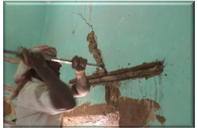
3. Filling the gap with wooden sticks.
