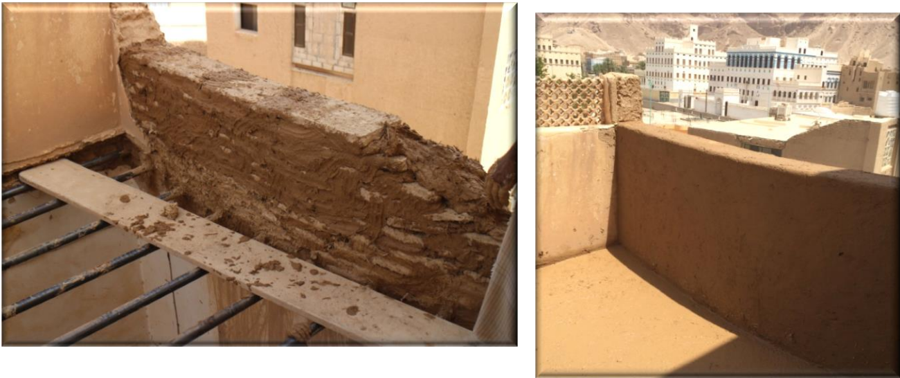
Figure 97. Before and after wall rebuild in al_Juniad house (Al-Aidarous,2014)
