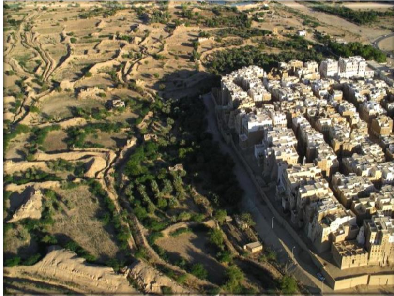
Figure 64. Site view of Shibam (Yehya)
