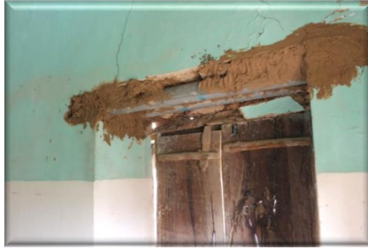
1. Replaced the structure element above the window (a steel stick)
