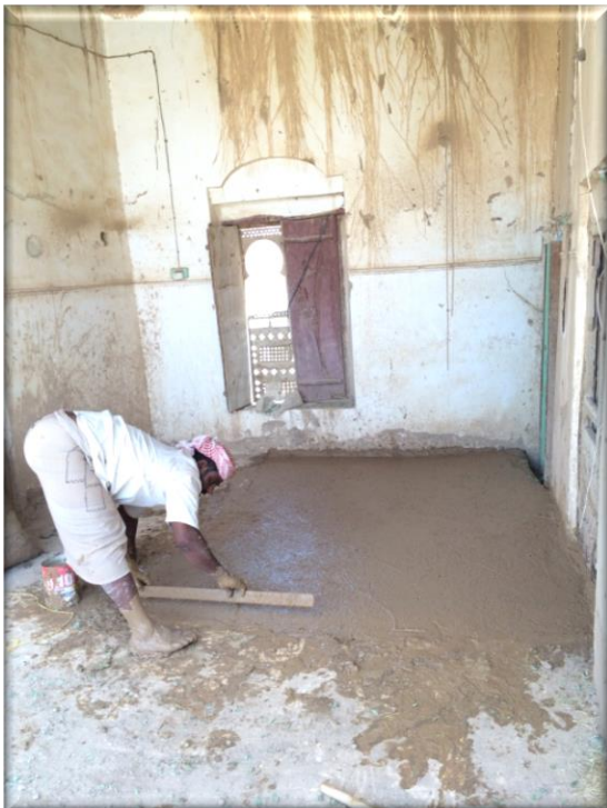
Figure 98. Restoration process of Al-Junaid house roof slabs (Al-Aidarous,2014)
