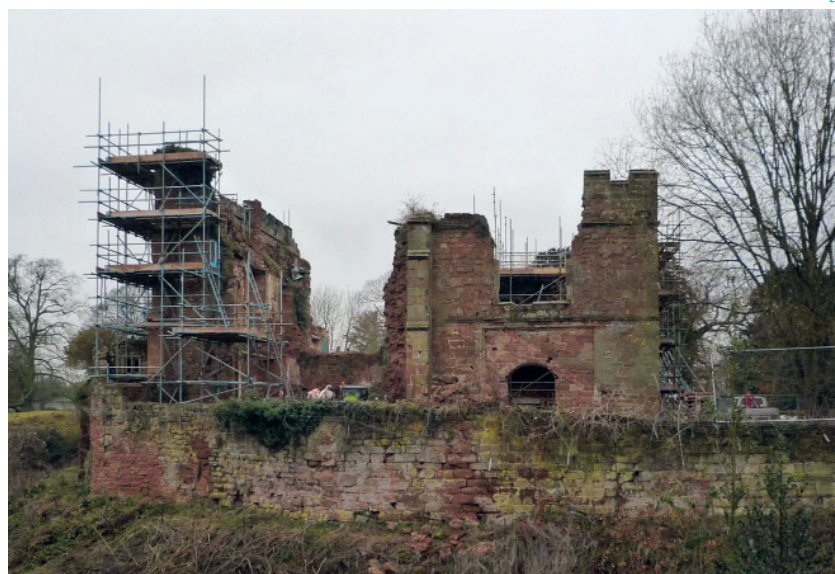
4. Vista del muro oeste previa a la restauración, 2007 4. As found: looking up the West wall, 2007
