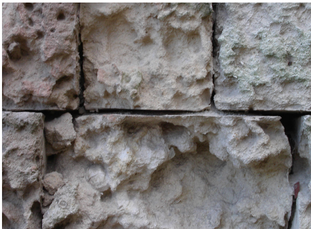
Figure 6. Alveolization of calcarenite
