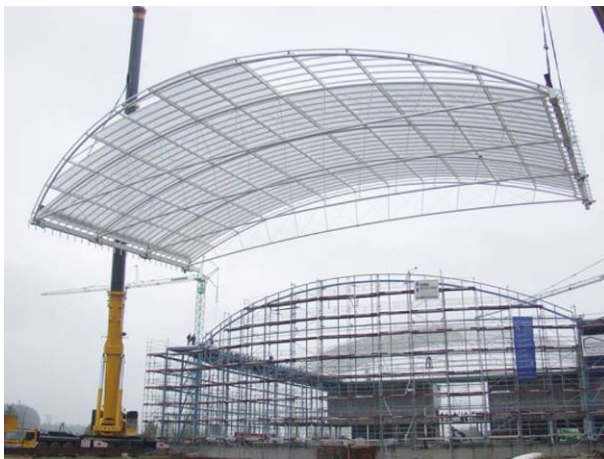
Figure 7: Half preassembled roof placed into position by two truck mounted cranes
