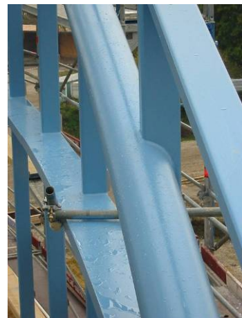
Figure 8: Upper detail of façade
