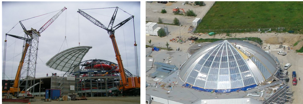
Figure 13: Roof of water slide paradise in Erding
