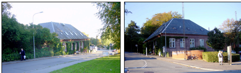
Figure 1: Existing porters lodge from (a) Northwest, and (b) Southwest
