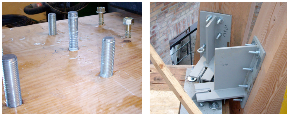
Figure 6: (a) Test of glued anchors, and (b) beam-column connections
