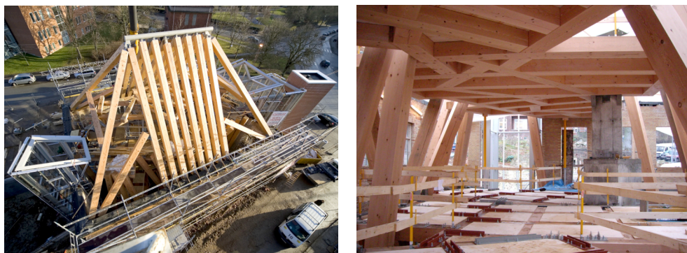
Figure 4: Structure under erection (a) Roof structure, and (b) Ground level
