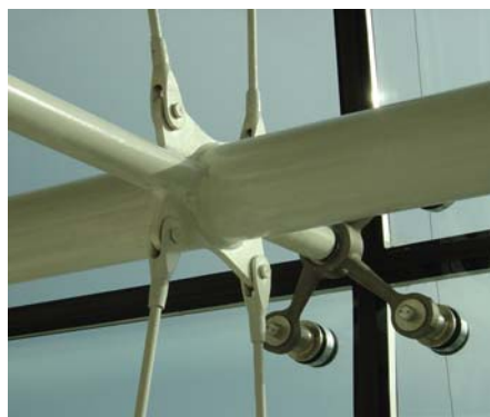
Figure 12: Tension rods to bow-truss
