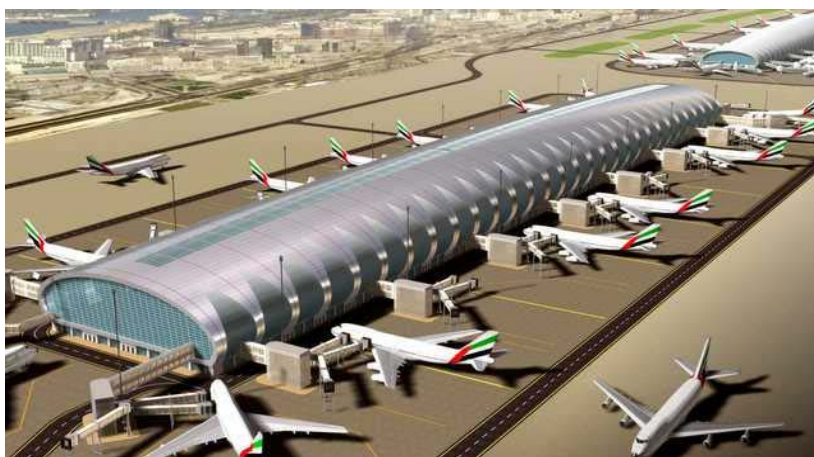
Figure 1: Expansion of Dubai International Airport (Concourse 3 and Concourse 2)
