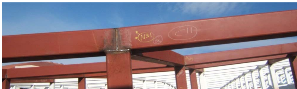
Figure 11. Welding control testing.
