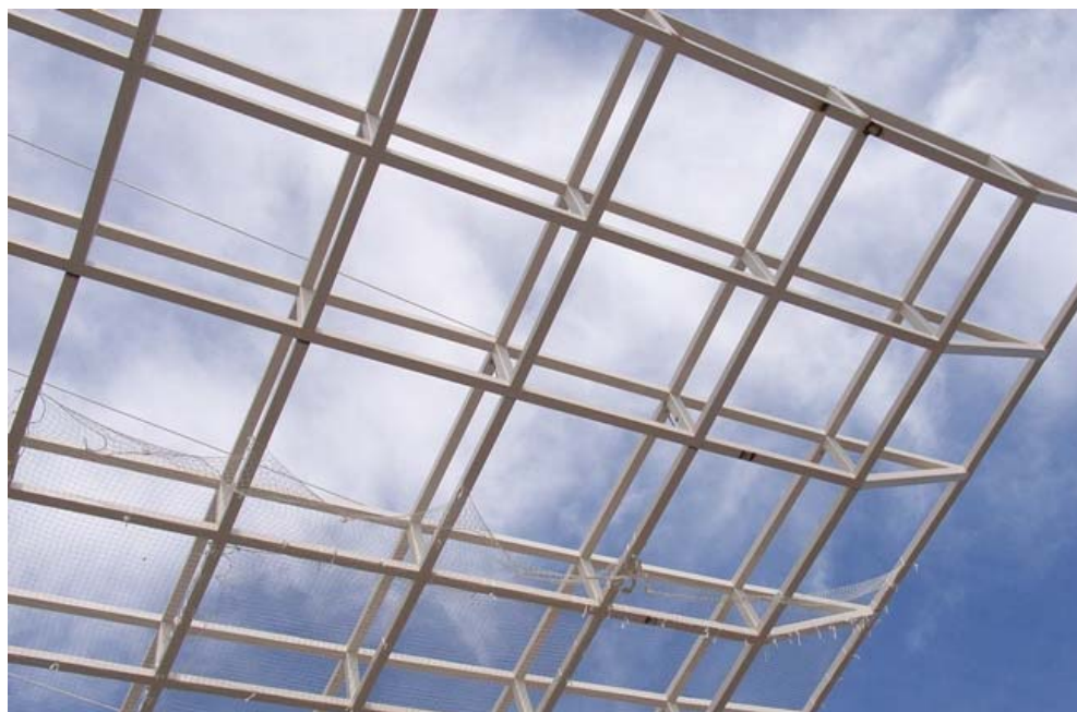
Figure 14. Aspect of the complete structure.
