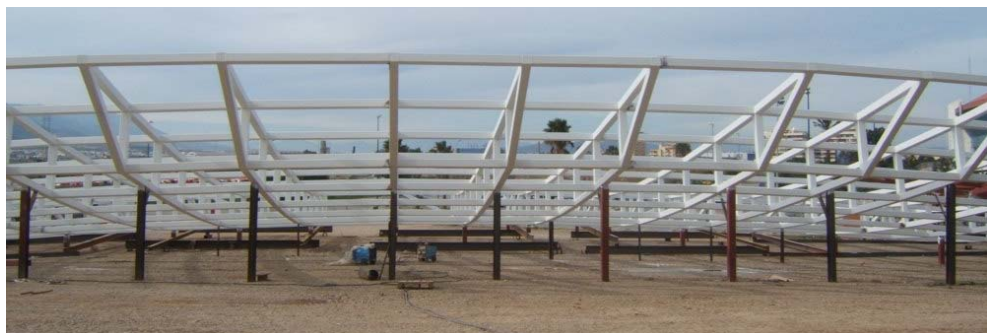
Figure 12. Prior assembly of the entire structure on the ground.
