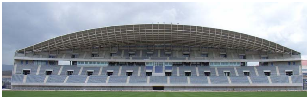
Figure 16. General view of the complete finished roof.
