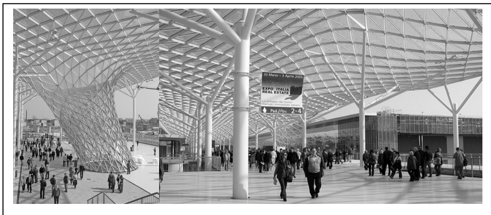
Figure 2: The Nuovo Polo Fiera Milano (Italy 2004, architect Fukas in collaboration with Schlaich Bergermann und Partner and Mero & co) illustrates how the architectural shell is discretised in quad angulated and triangulated (at the supports) meshes.
