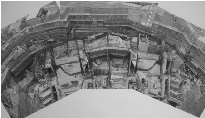
Fig.22 Formwork of the audience seat and radial girders
