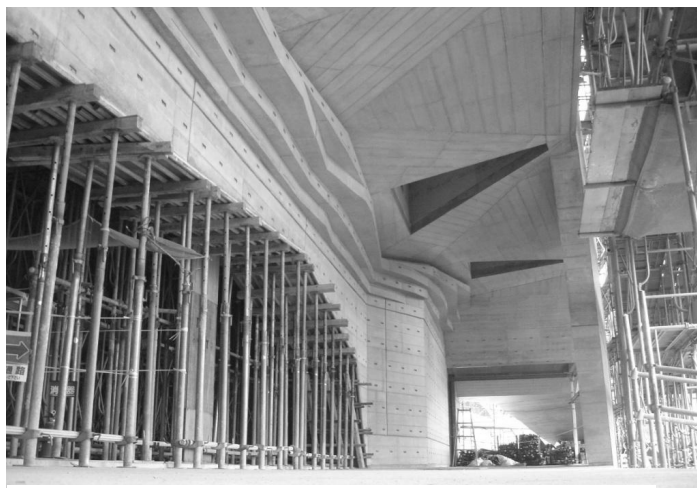
Fig.21 Temporary supports under the hall, 1 st floor level
