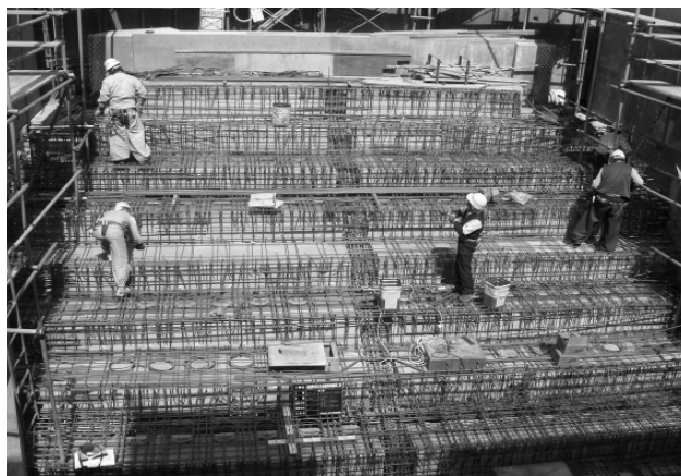
Fig.23 Reinforcement of the audience seats and girders
