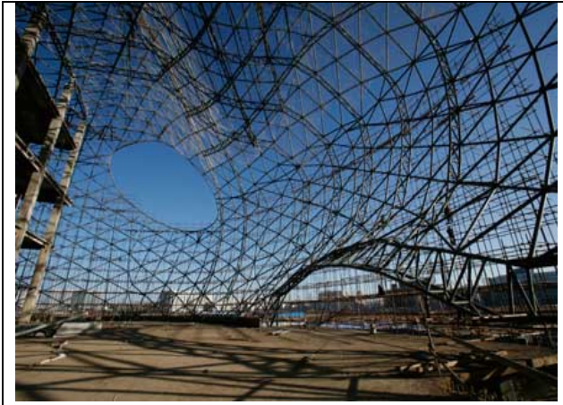
Fig.8 Detail of the structure under construction
