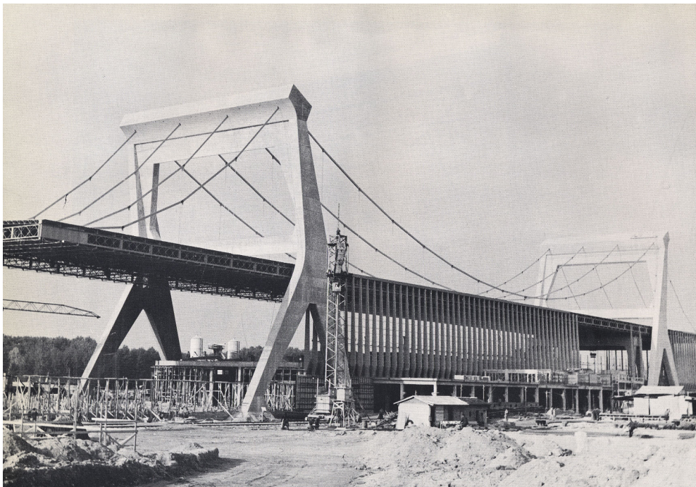
Figure 7. The Burgo Paper Mill in construction [MAXXI]
