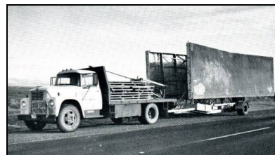
Figure 3: Prefabricated Umbrella Forms in Transit (photographs courtesy of Jack Christiansen)
