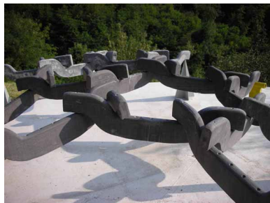
Figure 8. The assembly of a temporary structure composed of twenty-five reciprocal “short beams” interconnected according to the Fullerian geodetic scheme (a pentagon formed of five hexagons).
