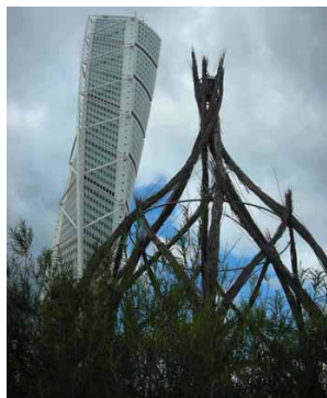
Figure 13. Santiago Calatrava: the Turning Torso skyscraper and the reconstruction of a Scandinavian aboriginal construction based on the static principle of the “spatial reciprocal structure”, Malmö - Sweden, 2005.
