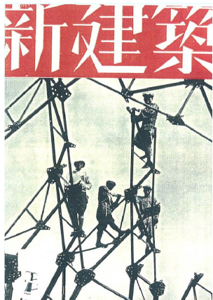
Photo 1: Diamond Truss under erection, from 'SINKENTIKU' (1936)
