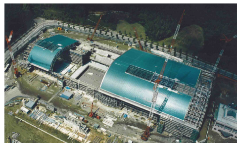
Photo 7: Sliding method with temporary cables, Suzuka Swimming Pool (1996)
