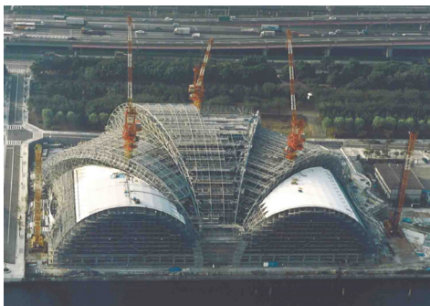
Photo 3: Element erection method, using full-scaffold, Tatsumi Swimming Pool (1993)
