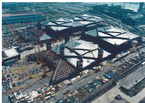
Photo 9: Lift-up method, East Exhibition Hall of Tokyo Big Sight (1994)
