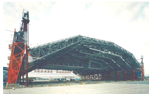
Photo 10: Lift-up method with temporary wires, ANA Osaka Overhaul Hangar (1987)
