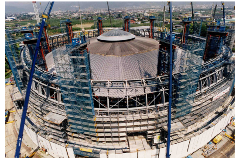
Photo 11: Lift-up method with temporary wires and a ring, White Rink (1995)
