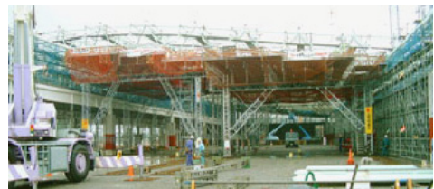
Photo 6: Move-scaffold method, Koriyama Wholesale Market (1999)
