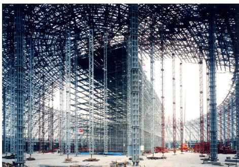
Photo 5: Block erection method, using temporary supports, Shiga Pref. Nagahama Dome (1991)
