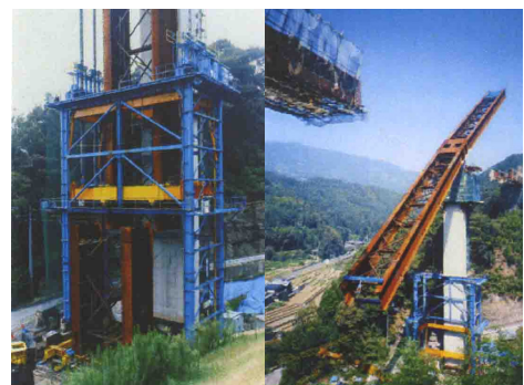
Photo 12: Jack-up turn method, Sukumo Viaduct (1999)
