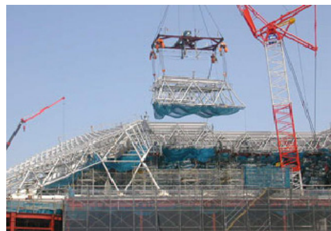
Photo 4: Block erection method, using temporary supports, Sky-Hall Toyota (2006)
