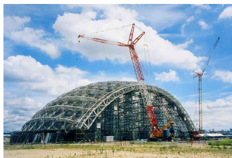
Photo 13: Jack-down with tie-beam, Okayama Dome (2002)
