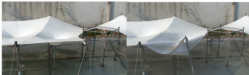
Breaking of cable No.48
