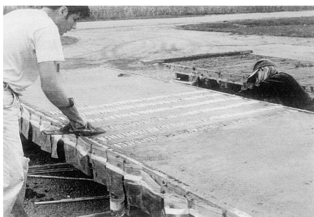
Fig. 2-38 – Glass tubes in a bridge deck (Dry, 2000).
