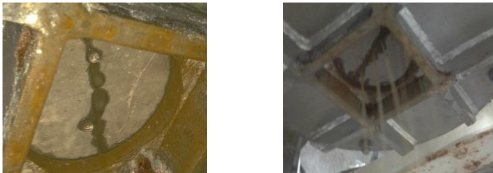
Fig. 3-14 – Inferior part of an specimen during the permeability test showing water flow for a small crack (left) and a large crack (right).
