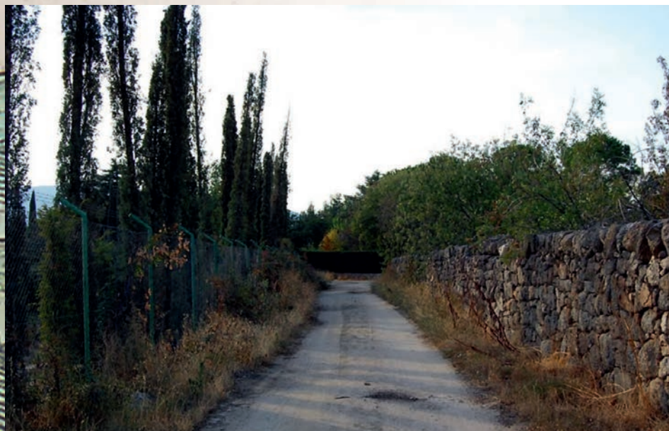
6. Dry masonry walls of the 16th century boundaries in El Escorial; East part beside the Medieval hamlet of Navalquejigo (Picture by the author).
