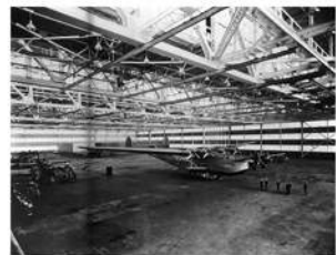
Fig. 17 Albert Kahn. Assembly Building, Glenn L.Martin Company Plant, Baltimore.
