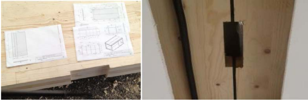
Fig. 12. Groove in joint between modules.
