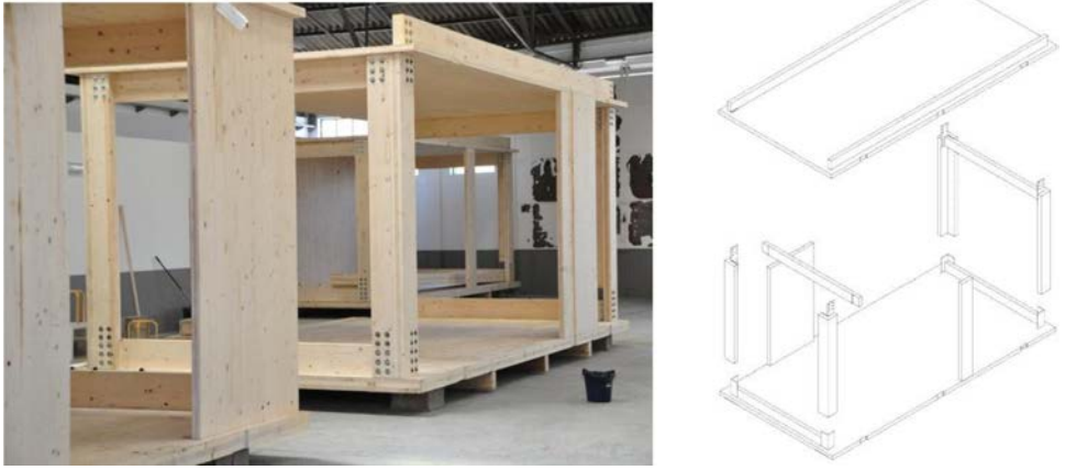
Fig. 3. Structural base module.
