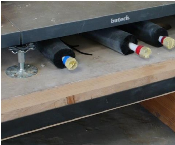
Fig. 13. Neoprene band on the bottom seal.
