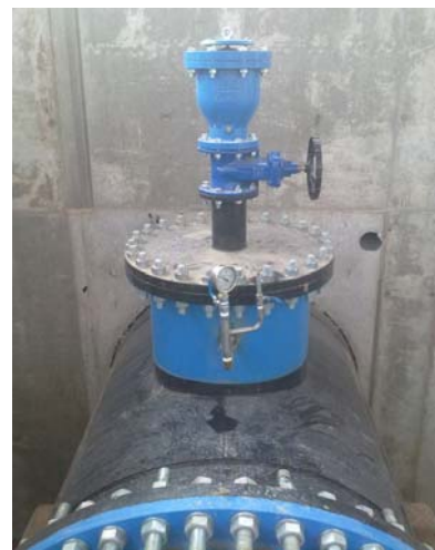
Figure 6. Air suction valve.
