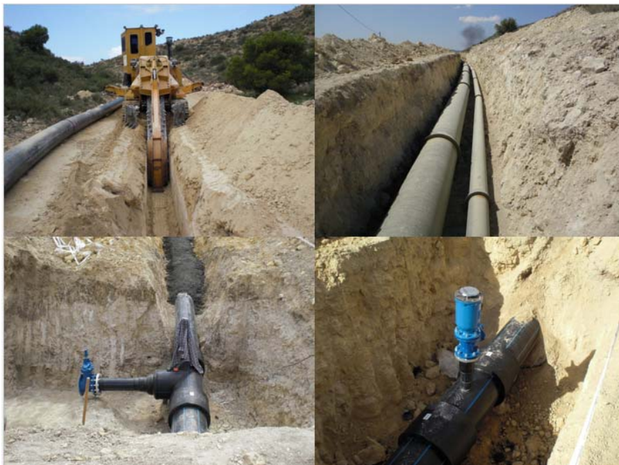
Figure 3. Construction of pipe ditches.
