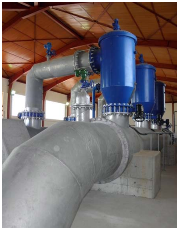
Figure 4. Installation of filters to avoid the networks' obstruction.
