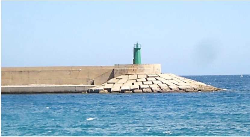
Figure IV.47. Uniformly-placed cube roundhead. Jávea, Alicante (Spain).
