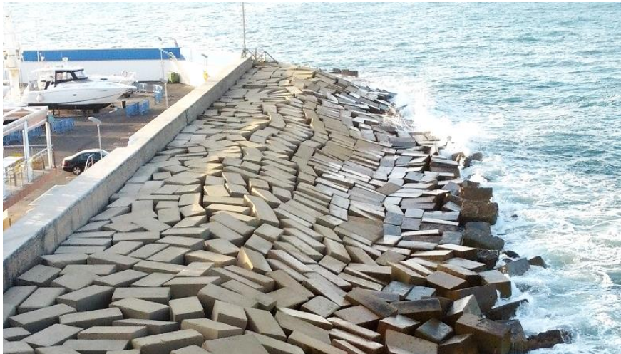
Figure IV.46. Double-layer armor with face-to-face fitting parallelepiped blocks. Mazarrón, Murcia (Spain).
