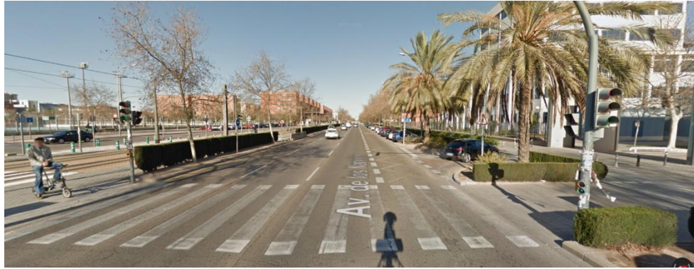
Figure 2- Photograph of Avenida de los Naranjos: it has a section of 70 meters, with 4 traffic lanes in each direction and a tram lane in the middle. Source: Google Street View (accessed on 20 th October 2014).
