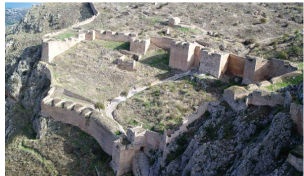
Figure 1: Aerial view of the survey area between the two defense lines, photographer: K. Xenikakis.
