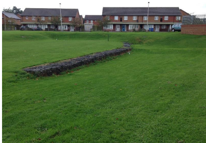
Figure 5. Infiltration basin implemented in Ardler, Scotland. (Photo taken by Ignacio Andrés Doménech).
