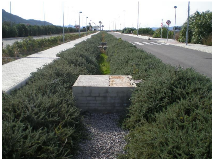
Figure 7. Green swale implemented in Xàtiva, Spain. (Photo taken by Ignacio Andrés Doménech).
