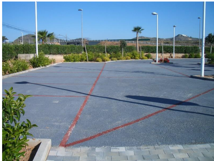
Figure 3. Permeable pavement implemented in Benaguasil, Spain. (Photo taken by Ignacio Andrés Doménech).
