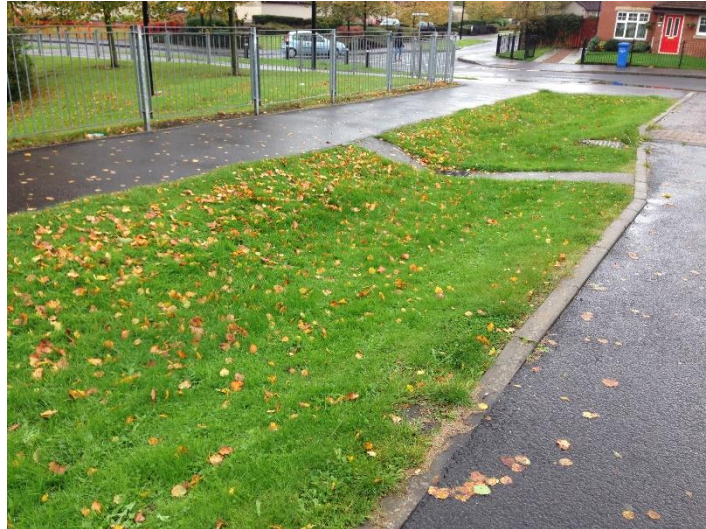
Figure 6. Green swale implemented in Ardler, Scotland. (Photo taken by Ignacio Andrés Doménech).
