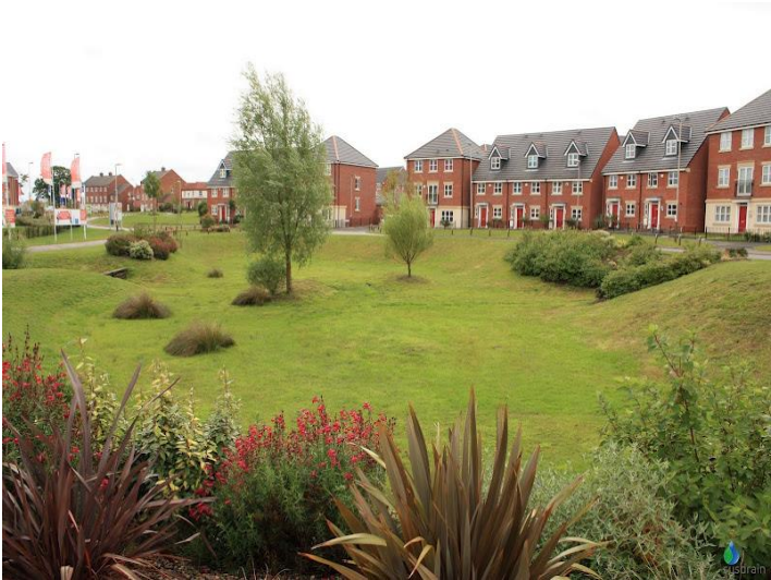
Figure 8. Detention basin. (Photo source: www.susdrain.org ).
