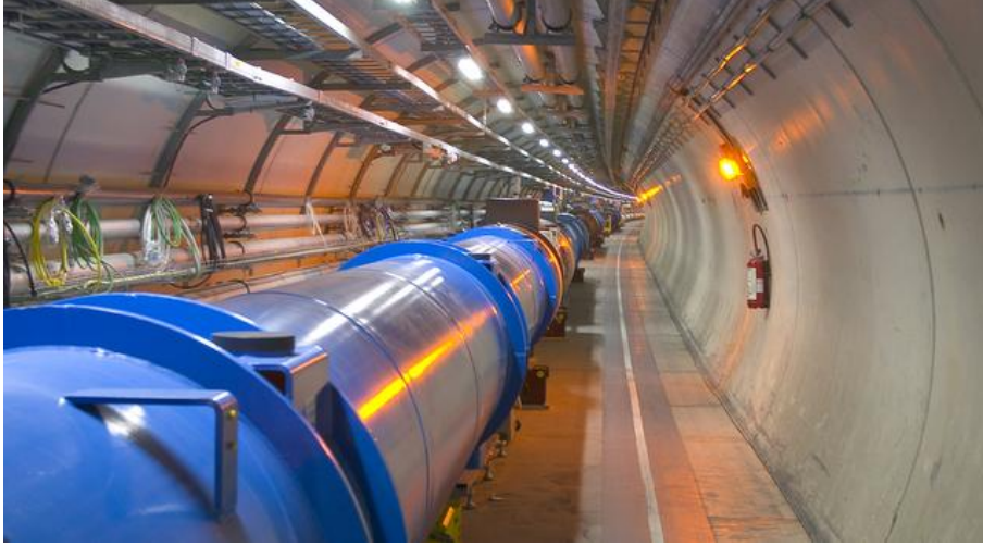
Figure 1.4: Picture of the LHC tunnel [5].
