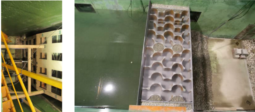
Figure 6. Absence of water leakages: a) wave paddle with interior face completely dry (left), b) model of the cyes-R with water on the left and dry (right).
