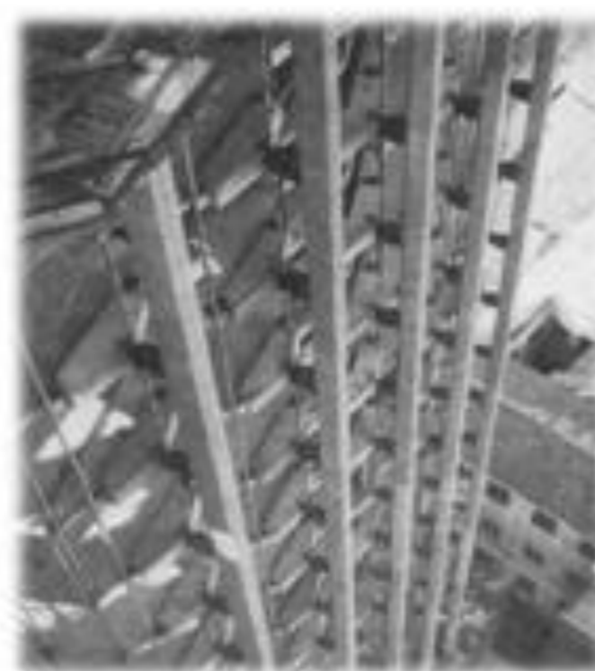
14. Joining the tie rods to the forged type
