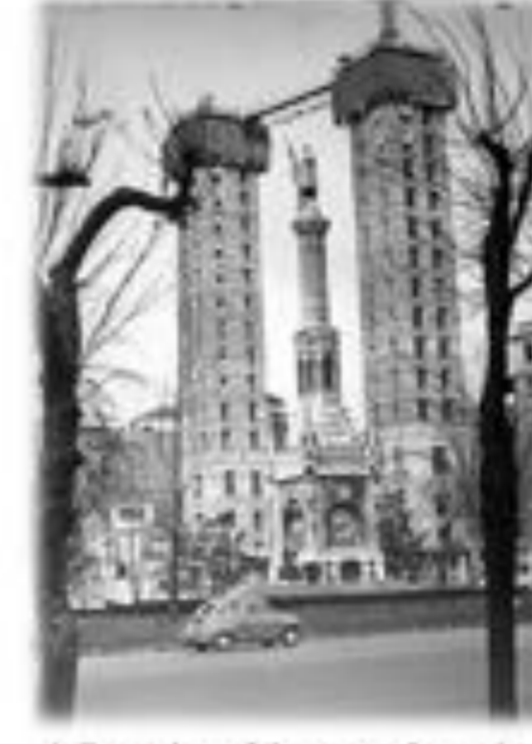
4. Execution of the central core in "Torres de Colón"
