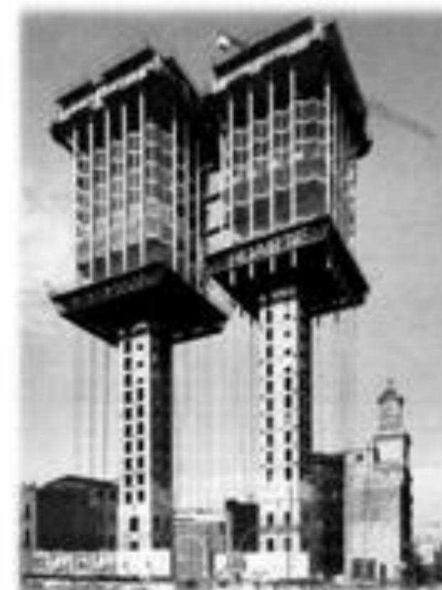
9. Execution of the slabs two by two
