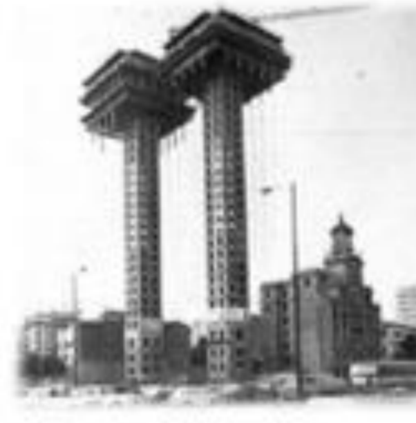
8. Execution of the head of the towers
