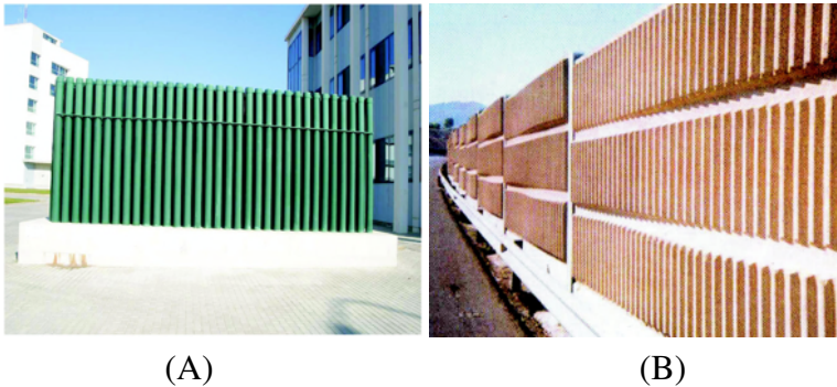
Figure 4.1: (A) SC used as acoustic barrier; (B) Classical acoustic barrier.
