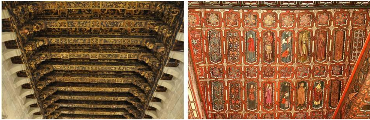
Figure 6.1.4. Coffered ceilings from Cámara de Dorado del Consulado del Mar la Lonja de Seda, Valencia 15th – 16th centuries (left) and Mudejar roof from Teruel Cathedral, 14th century (right).
