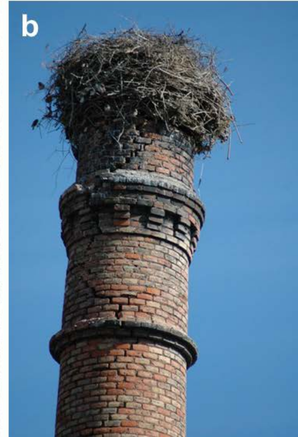
Fig. 16. a) Chimney in Catarroja (Spain) with mortar affected by the presence of insects; b) Chimney in Puertollano (Spain) weighed down by a large storks' nest in the crown.
