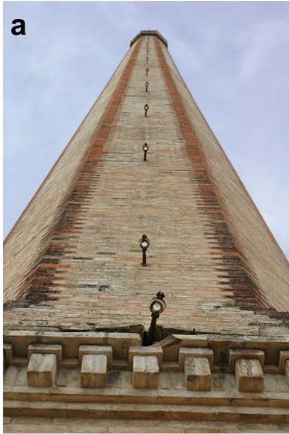
Fig. 7. Damage caused by corrosion of metal components in a chimney in Gandía (Valencia): a) General view; b) Close-up.
