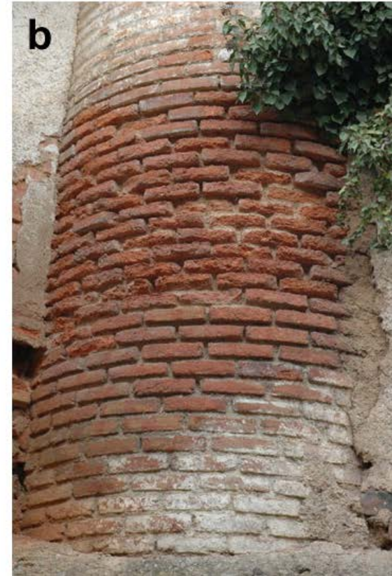
Fig. 3. Damage to bricks: a) Flaking bricks in a chimney in Peñarroya-Pueblonuevo (Spain); b) Efflorescence in a chimney in Daroca (Spain).
