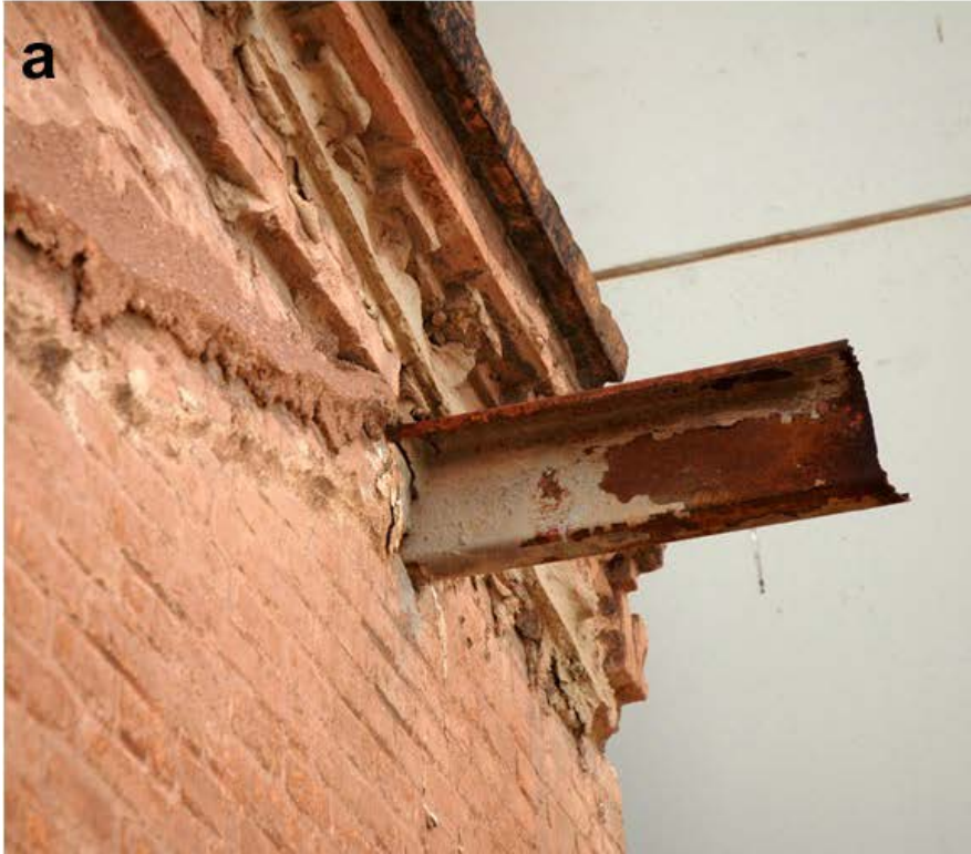
Fig. 18. a) Damage due to having to previously support an auxiliary structure in Foios (Spain); b) Grafitti on a chimney in Villaluenga (Spain).
