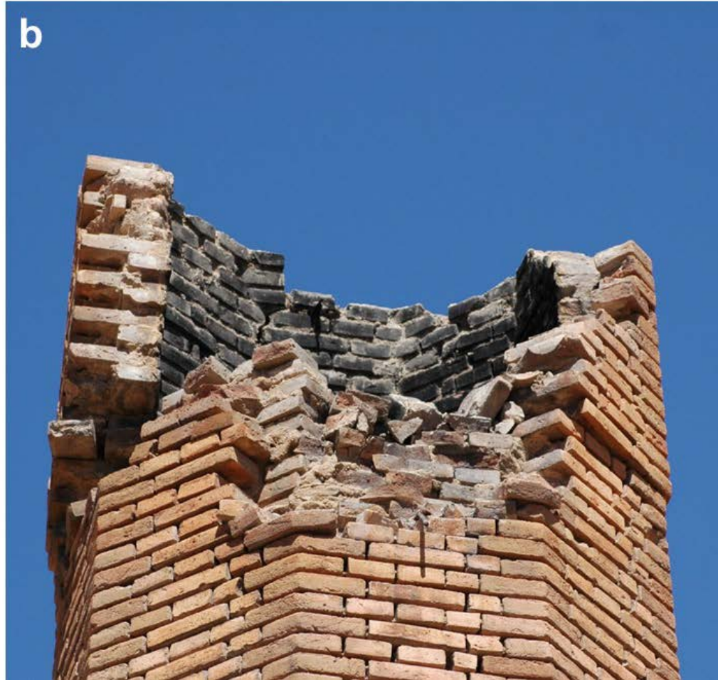
Fig. 12. Chimney in Villar del Arzobispo (Spain), part of which collapsed due to strong wind gusts: a) General view; b) Close-up.
