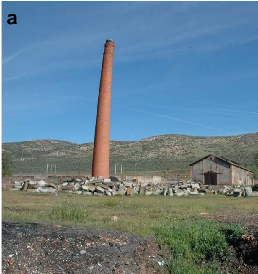
Fig. 8. Displacements caused by prevailing winds: a) Chimney in Puertollano (Spain); b) Chimney in Oliva (Spain) with large openings in stack and crown.
