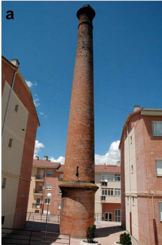
Fig. 10. Smoke stains on the upper section of a chimney in Segovia (Spain): a) General view; b) Detail of crown.
