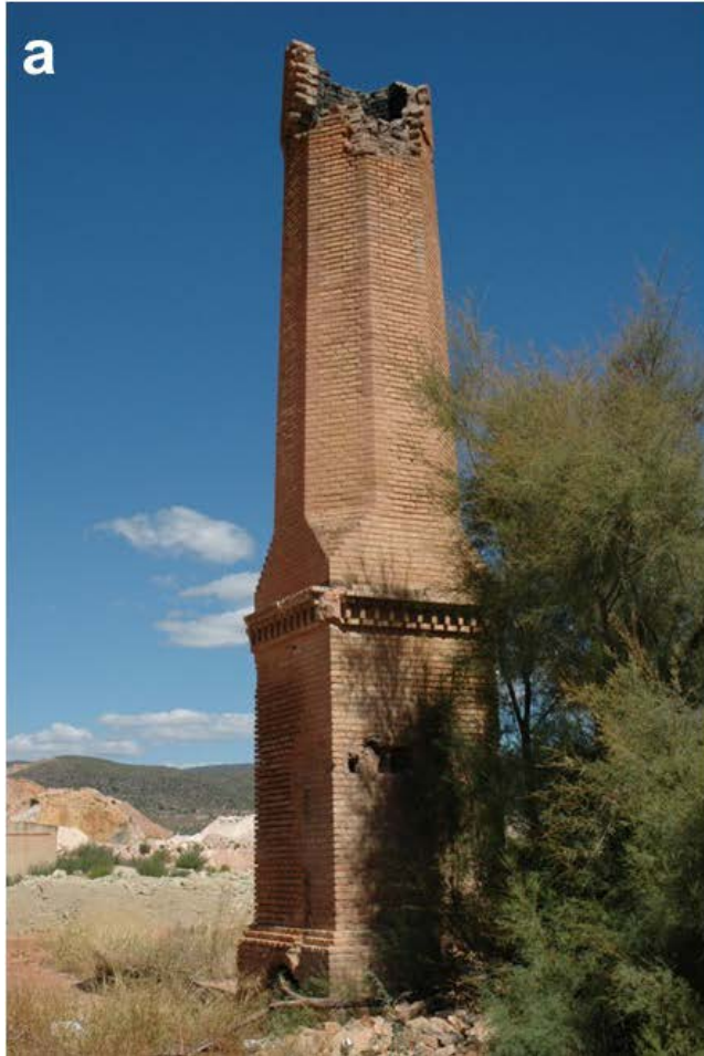
Fig. 12. Chimney in Villar del Arzobispo (Spain), part of which collapsed due to strong wind gusts: a) General view; b) Close-up.
