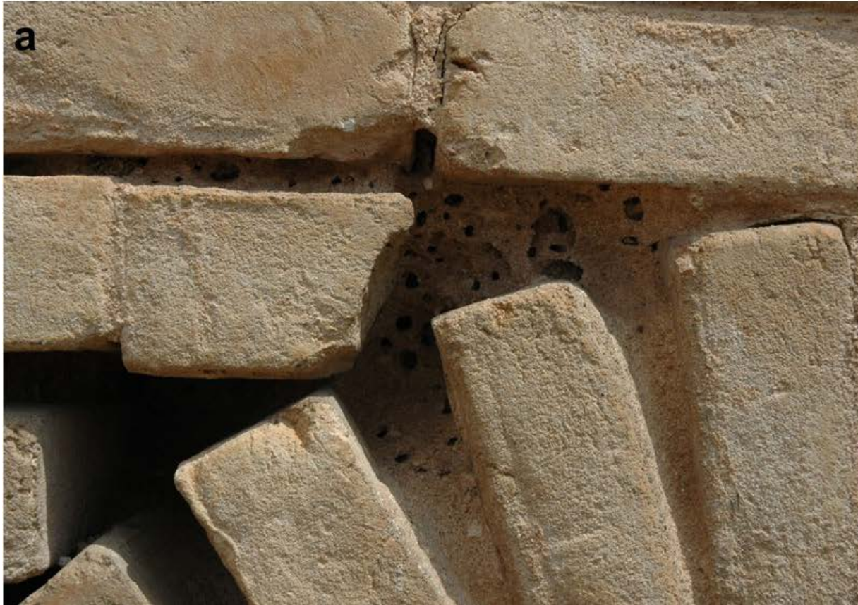
Fig. 16. a) Chimney in Catarroja (Spain) with mortar affected by the presence of insects; b) Chimney in Puertollano (Spain) weighed down by a large storks' nest in the crown.
