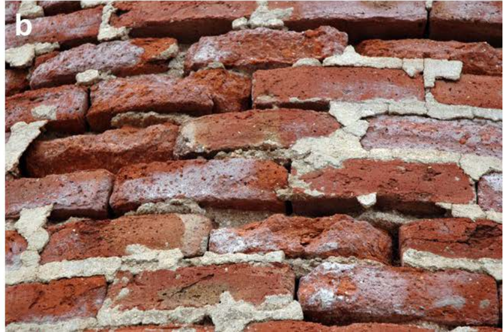
Fig. 5. Deterioration and missing mortar. Chimneys in: a) Manzanares (Spain); b) Cinco Casas (Spain).
