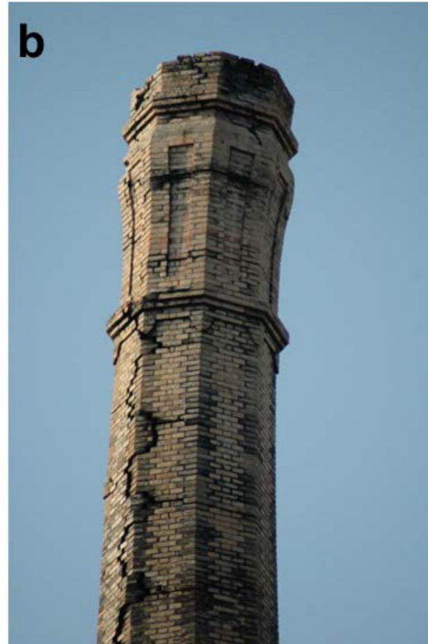
Fig. 8. Displacements caused by prevailing winds: a) Chimney in Puertollano (Spain); b) Chimney in Oliva (Spain) with large openings in stack and crown.
