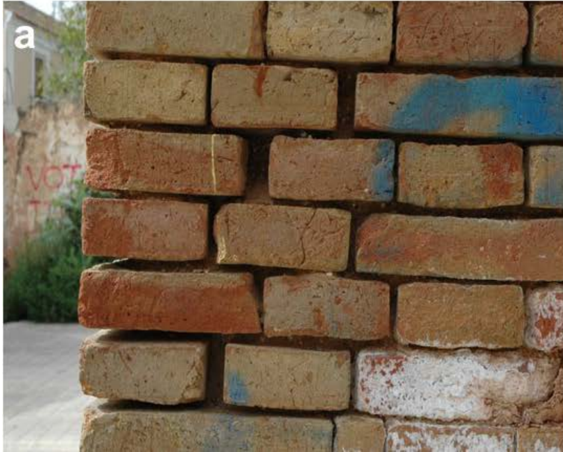
Fig. 5. Deterioration and missing mortar. Chimneys in: a) Manzanares (Spain); b) Cinco Casas (Spain).
