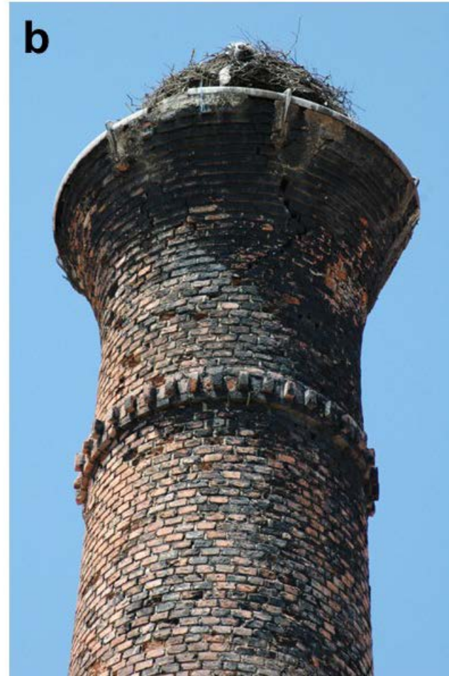
Fig. 10. Smoke stains on the upper section of a chimney in Segovia (Spain): a) General view; b) Detail of crown.
