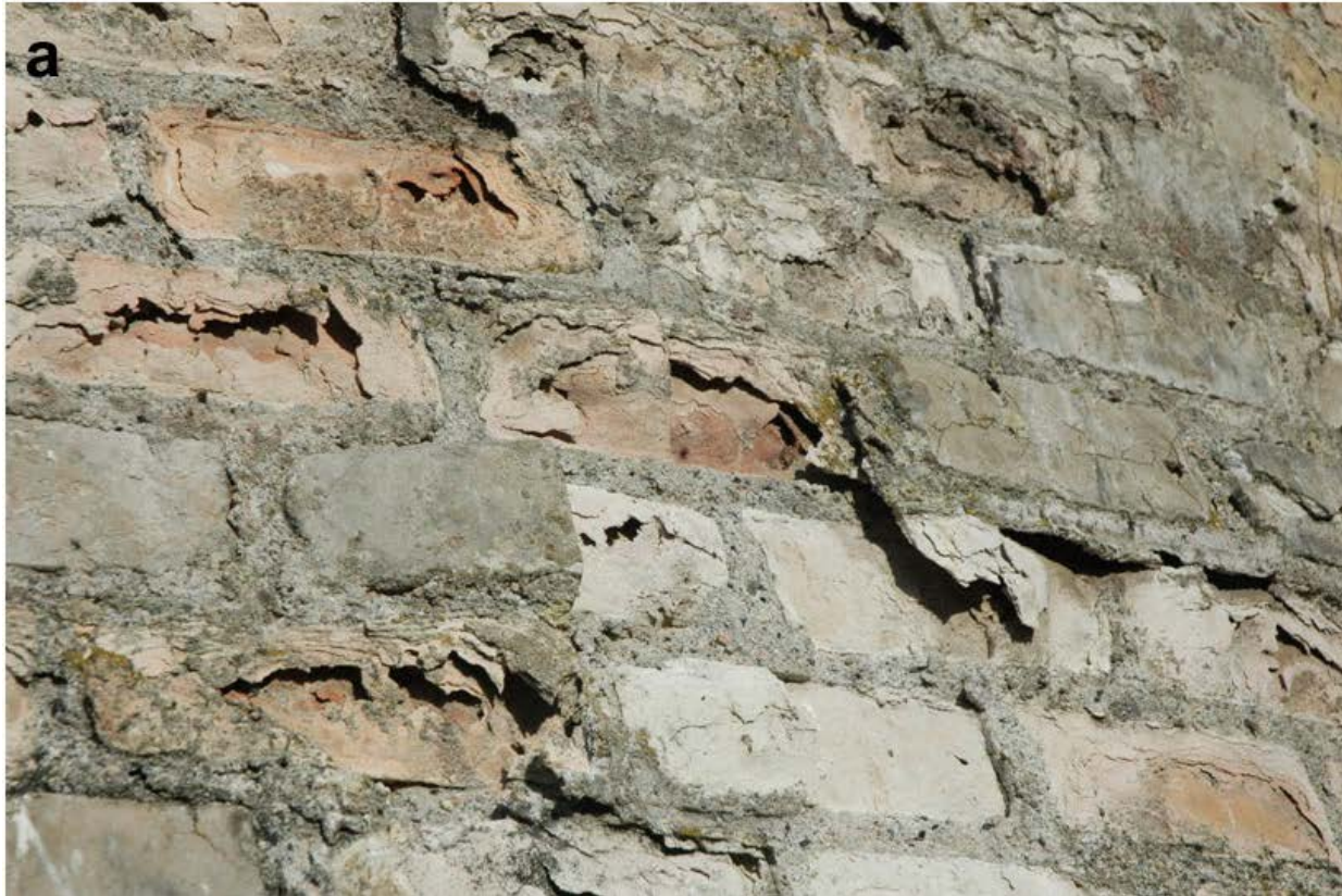
Fig. 3. Damage to bricks: a) Flaking bricks in a chimney in Peñarroya-Pueblonuevo (Spain); b) Efflorescence in a chimney in Daroca (Spain).
