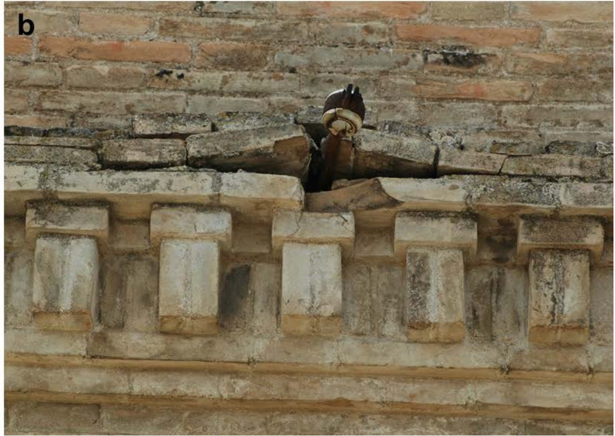
Fig. 7. Damage caused by corrosion of metal components in a chimney in Gandía (Valencia): a) General view; b) Close-up.
