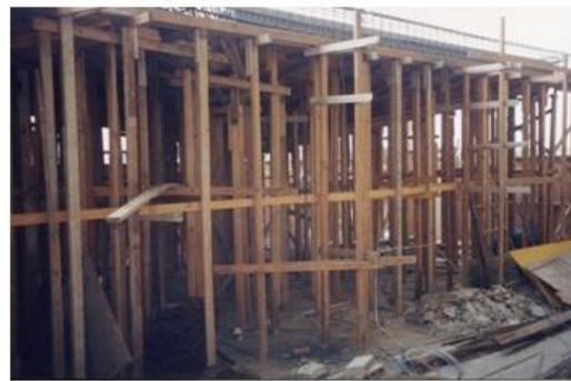
145 Fig. 3. Views of buildings supported by wooden shores: a) in Valencia (Spain) in the 1980s 146 and b) in El Calafate (Argentina) in the late 90s.
