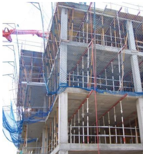
Fig. 2. Building under construction in Sabadell (Barcelona, Spain) in 2010 with three consecutively shored floors, two of which have been cleared and one is still completely shored.
