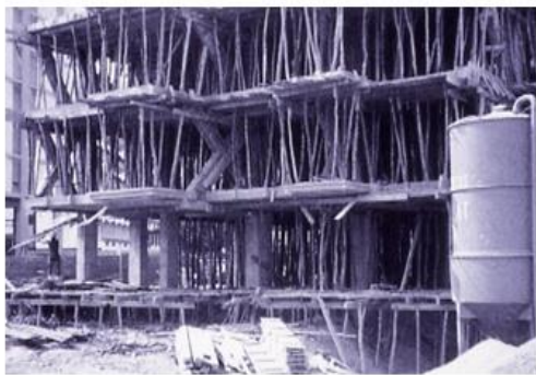
145 Fig. 3. Views of buildings supported by wooden shores: a) in Valencia (Spain) in the 1980s 146 and b) in El Calafate (Argentina) in the late 90s.
