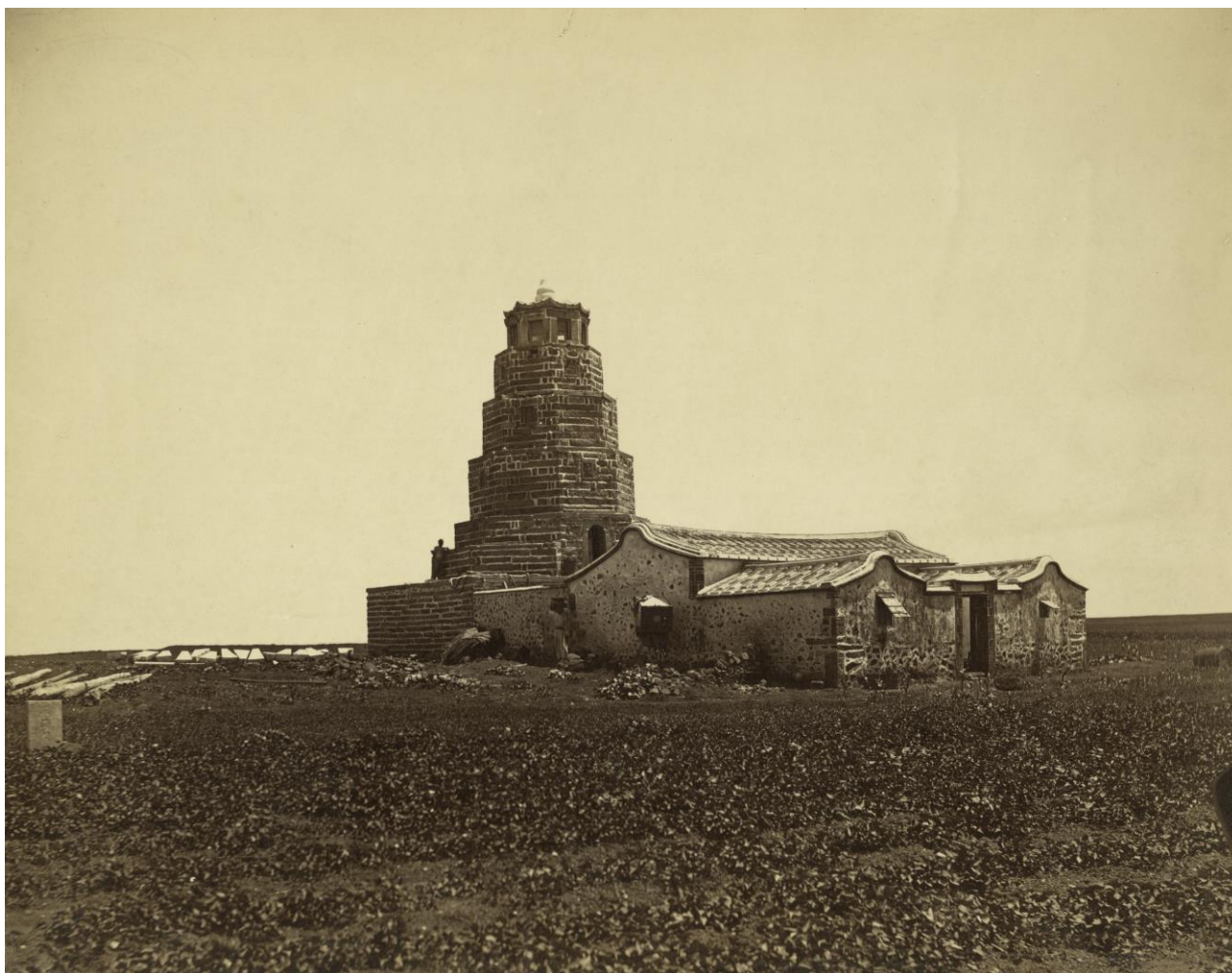
Figure 1: Xiyu Pagoda Lighthouse in a unique Chinese style demolished in 1875.
