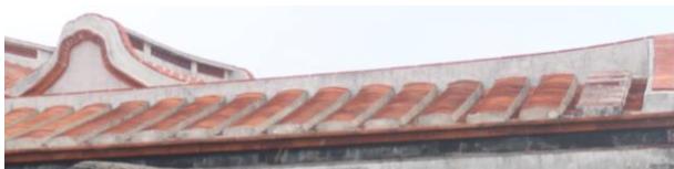
Figure 11: Existing yǎng hé tile in Erkan village.
