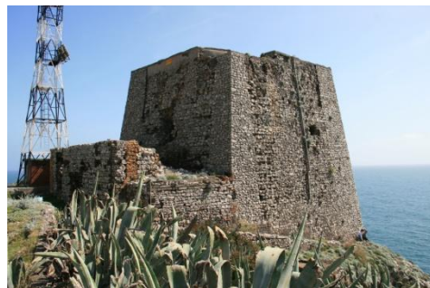
Fig. 3- Minerva Tower. The added structure on the northern side (2015)
