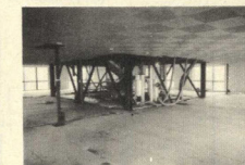
21 GEAI interior. Central circulation core and service stacks are fixed to structure. Floors are chipboard.
