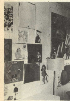
6 Carasso Internal movable steel faced partitions with magnetic picture hanging.
