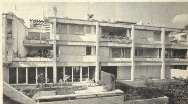
3 System 4D. External appearance at Zug reflecting the tastes and requirements of the residents. ( B & W 1/73)
