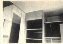
25 Västerås. Details of casework and partitions.
