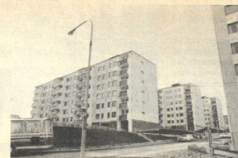
18 Tensta. Regimented layout on a difficult sloping site. Note balcony units that clip on to structural system.
