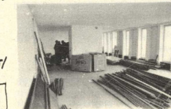
11 Flat before partitioning, showing moulded ply-trim in foreground and air-extract in core.
