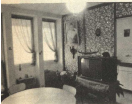
15 Informal living room adjoins kitchen. Note wallpapering between cover strips over partition joints.
