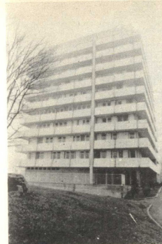
7 Montreaux. Note variation in facade resulting from occupants' choice of position of panels.
