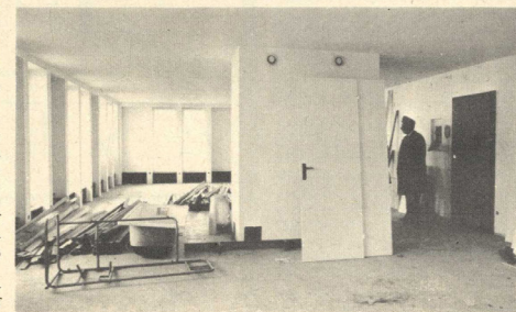
4 The essential flexibility II: the occupier now makes his choice of layout (GEA system, France).
