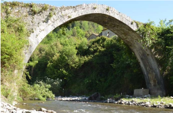
Figure 11: The Hannibal Bridge.
