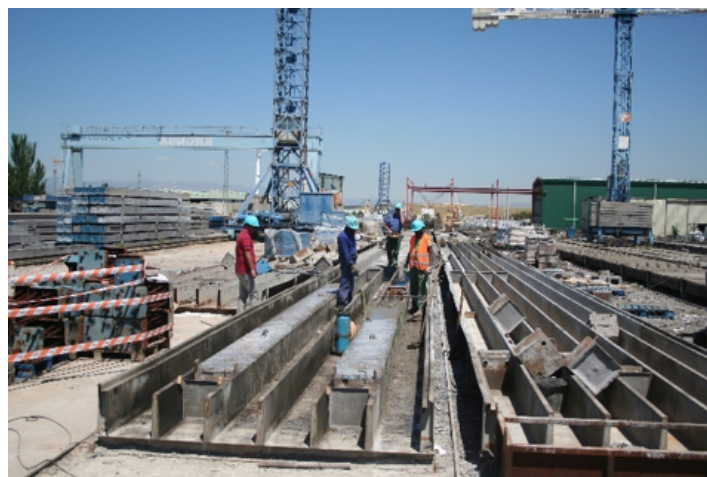
Figure 1. Precast pile at the factory Rodio-Kronsa
