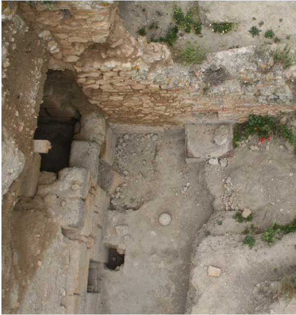
Fig. 5. North wall and Torre Menor meeting, currently hidden. PDA (2011).
