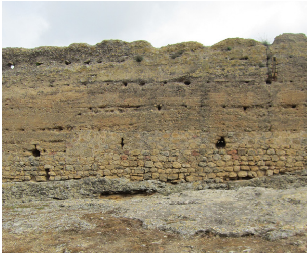
Fig. 13. Outer western wall with two types of embrasures: stick and orb-stick. Source: the authors.
