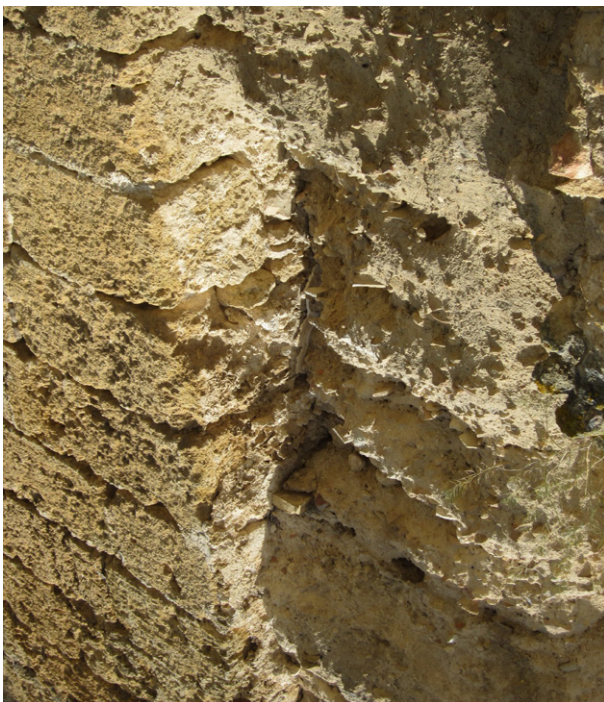
Fig. 11. Overlapping rammed earth and ashlar blocks with plaster between them. Source: the authors.
