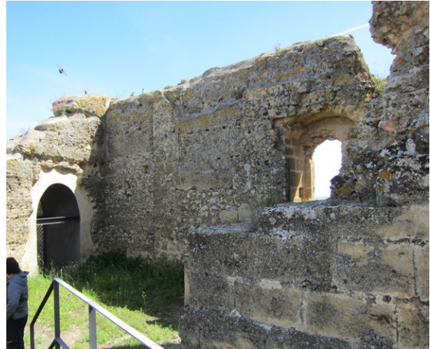
Fig. 14. North gate and postern gate with a discontinuity in the east wall. Source: the authors.
