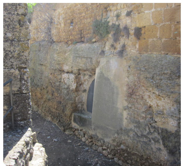
Fig. 16. Entrance to a cave excavated on the north side of the moat, used as a dwelling in the 20 th century. Source: the authors.
