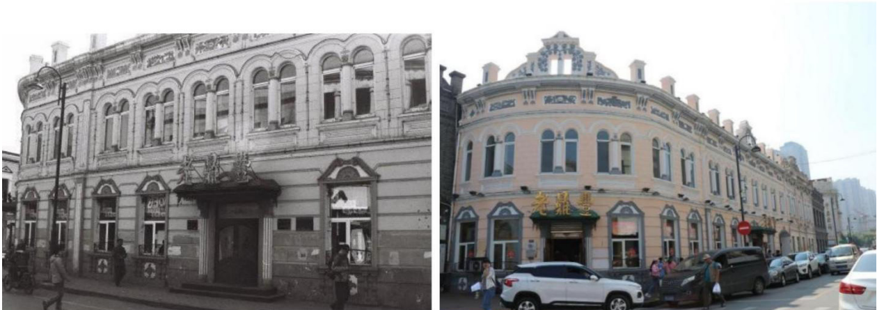
Fig. 12. Laodingfeng Building. Left: image from 2000 (Zhou Liting, 2018). Right: actual image (Author).
