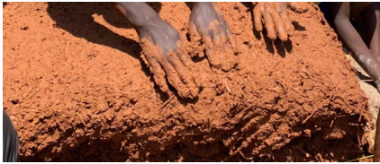
Fig. 5 – Cob building in process.
