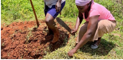
Fig. 4 – Preparation of Cob Mixture.
