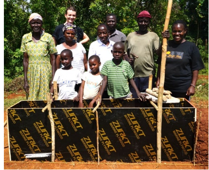
Fig. 6 – Group of rammed earth building process with finished framework.
