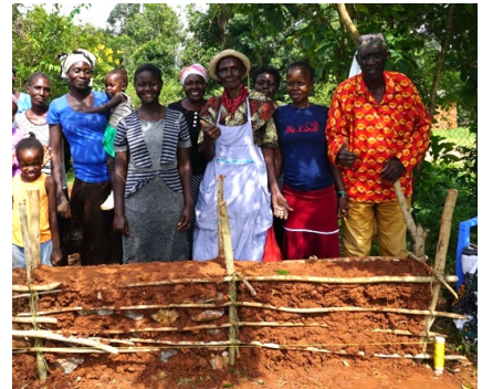
Fig. 3 – Wattle & Daub group with finished test wall.
