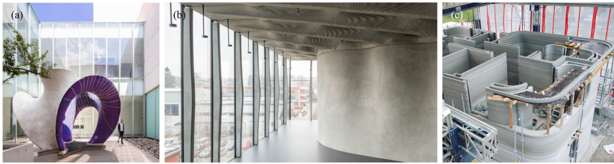
Fig. 1. Exemplary applications of digitally fabricated concrete: (a) KnitCandela concrete shell from [6] (Photo credits: Angelica Ibarra); (b) façade mullions produced with Smart Dynamic Casting [7], curved wall produced with the Mesh Mould Technology [8], and Smart Slab produced with a Particle-bed binding formwork [9] (Photo credits: Roman Keller); (c) construction of a house with 3D concrete printed walls in Germany (Photo credits: PERI).
