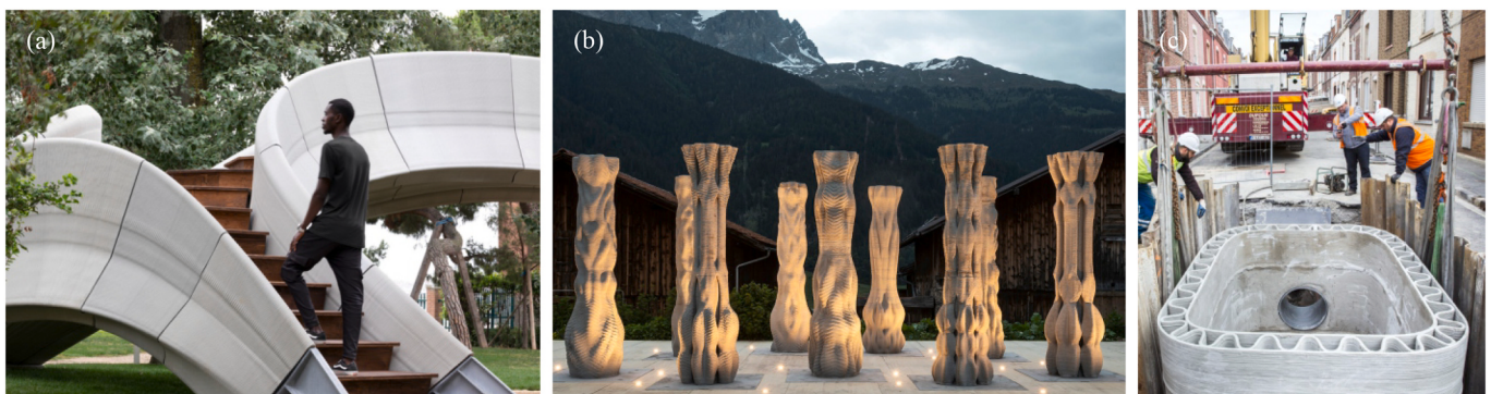
Fig. 6. Exemplary applications of 3DCP : (a) Striatum – 3DCP footbridge [40] (Photo credits: Studio NAARO); (b) 3DCP Concrete Choreography described in [41] (Photo credits: Benjamin Hofer); (c) 3DCP stormwater collector [42].
