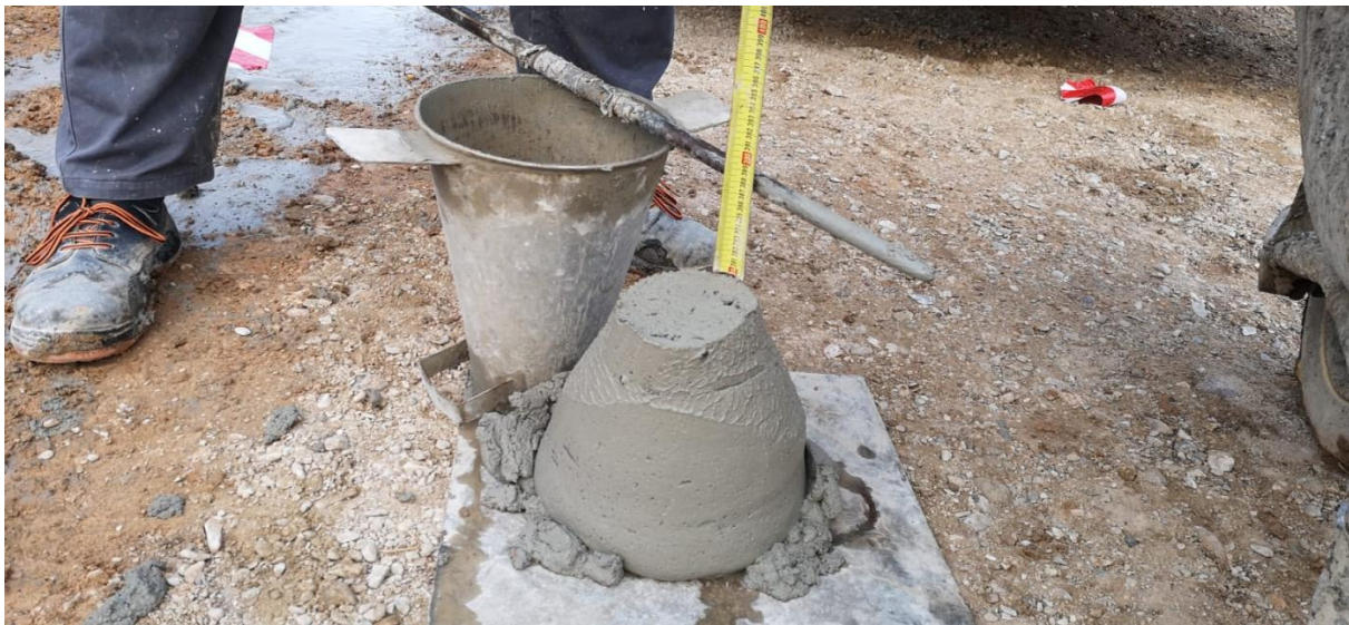
Figure 7. Control of the consistency of the mortar L.M. of Column no. 24. The Abrams cone gives values between 8 and 12 cm. The location of this column is shown in Figure 5.
