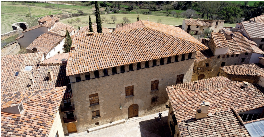
Figure 2. Aerial view of the survey site. 2022
