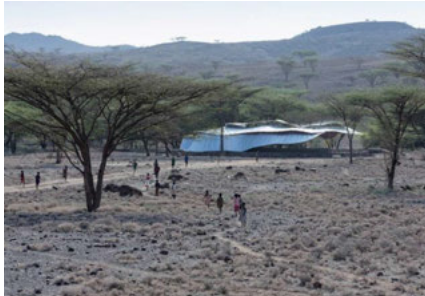
Figure 4. Konokono clinic in Turkana, Kenya © Iwan Baan Architects: Selgas Cano, Ignacio Peydro and students from MIT studio Unmaterial
